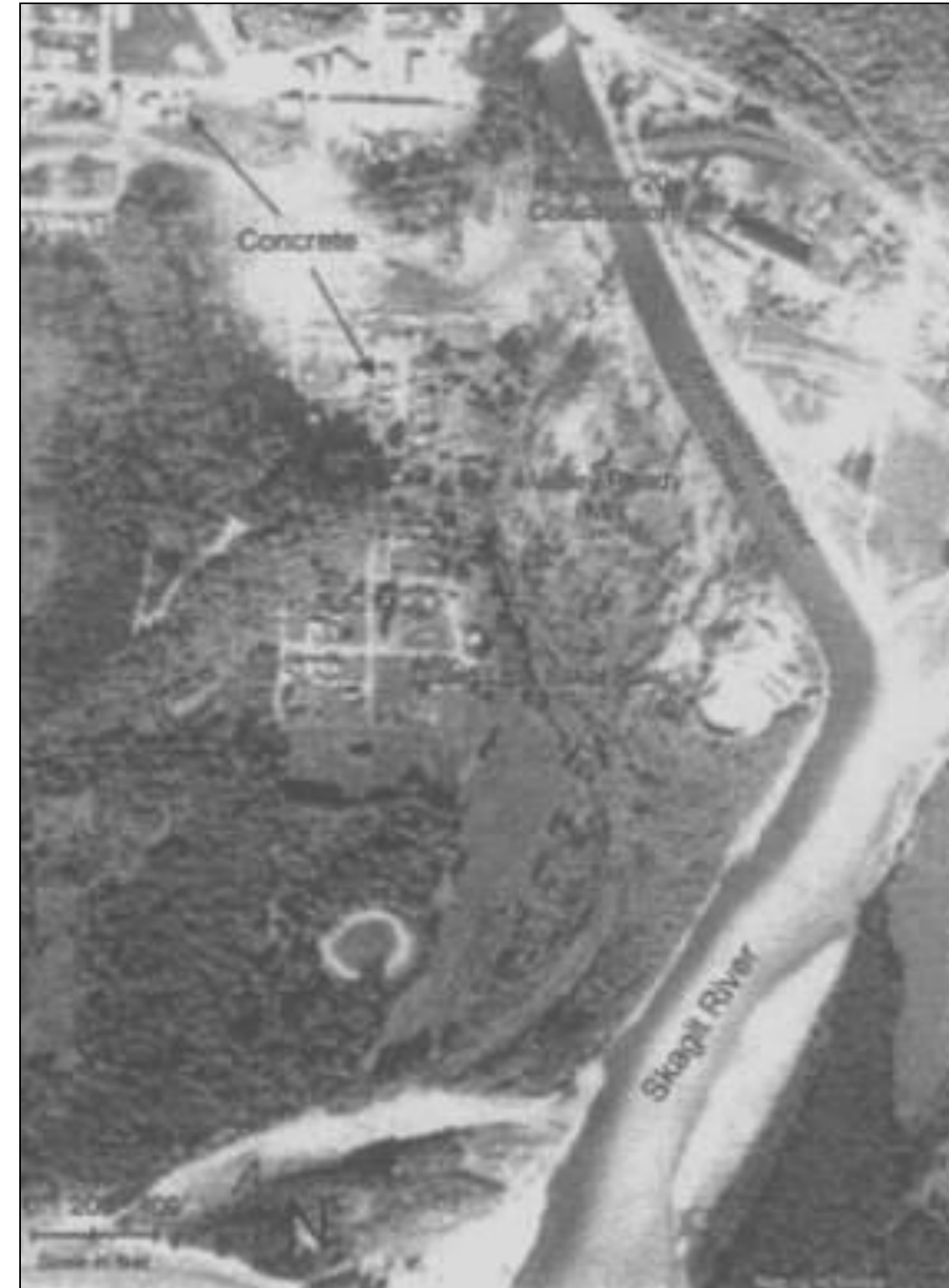
Baker River after dredging, circa 1967, showing the dried-up Little Baker former side channel.
