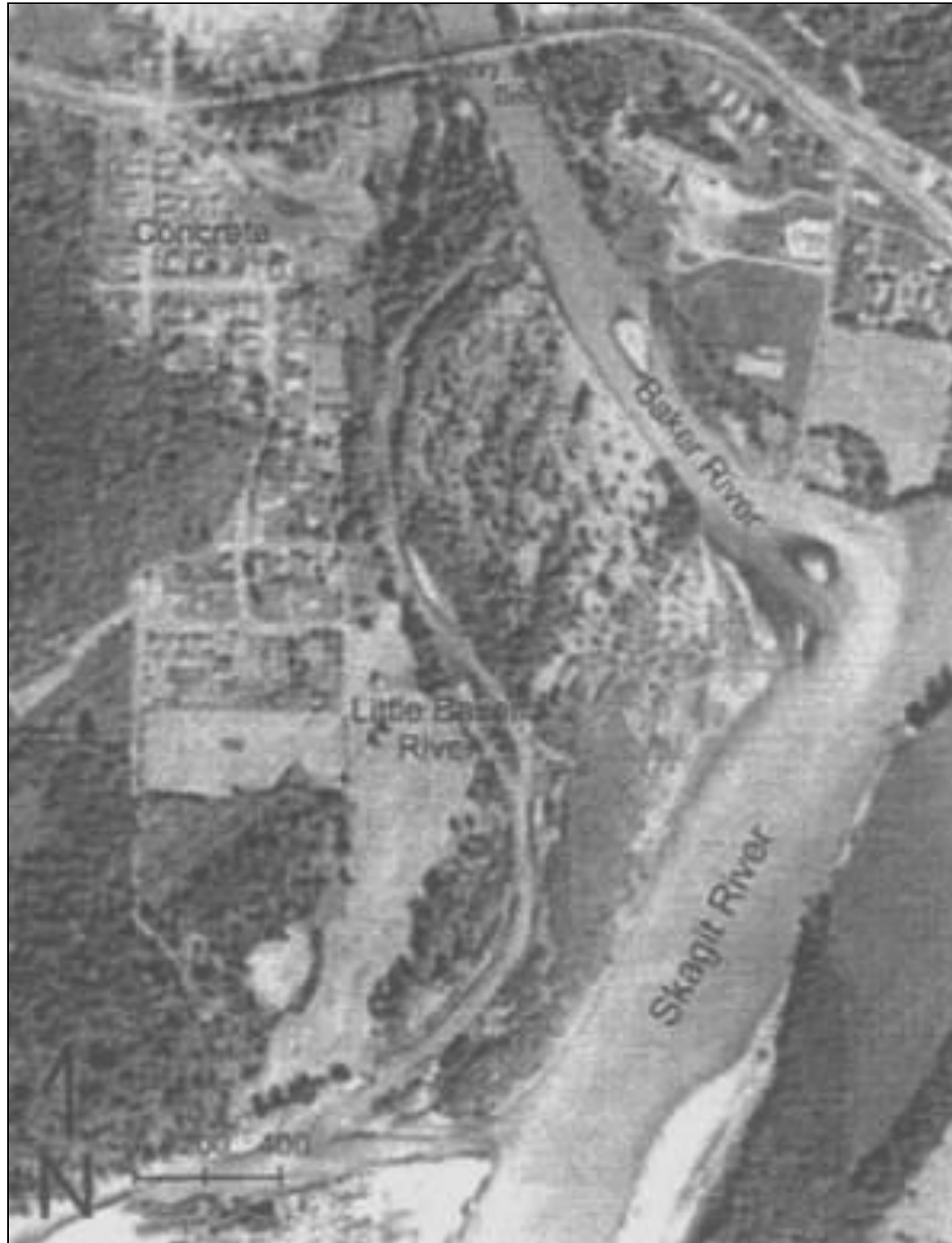
Historical view of the Baker River and Little Baker side channel circa 1956, prior to dredging of the Baker River.
