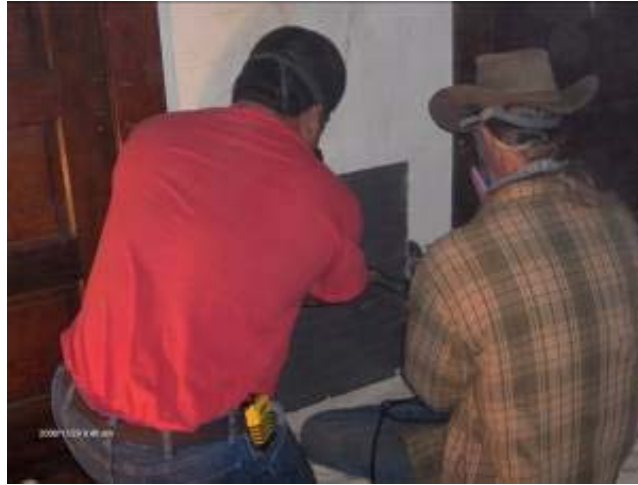
Graphic 6: Carpenters removing lath from wall. Wall has been duct-taped to preserve integrity of the plaster.
