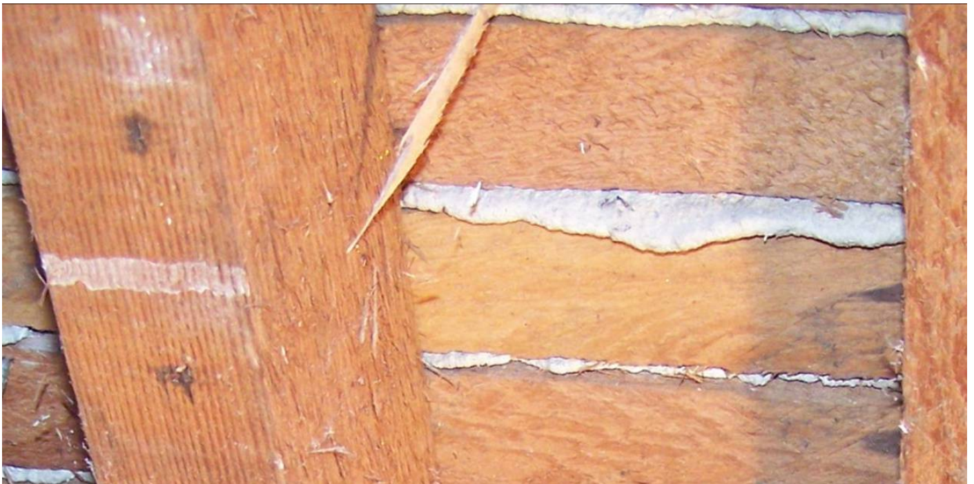
Graphic 9: Close-up of initial wall cutout. No bleaching or discoloration of the original lath was observed.
