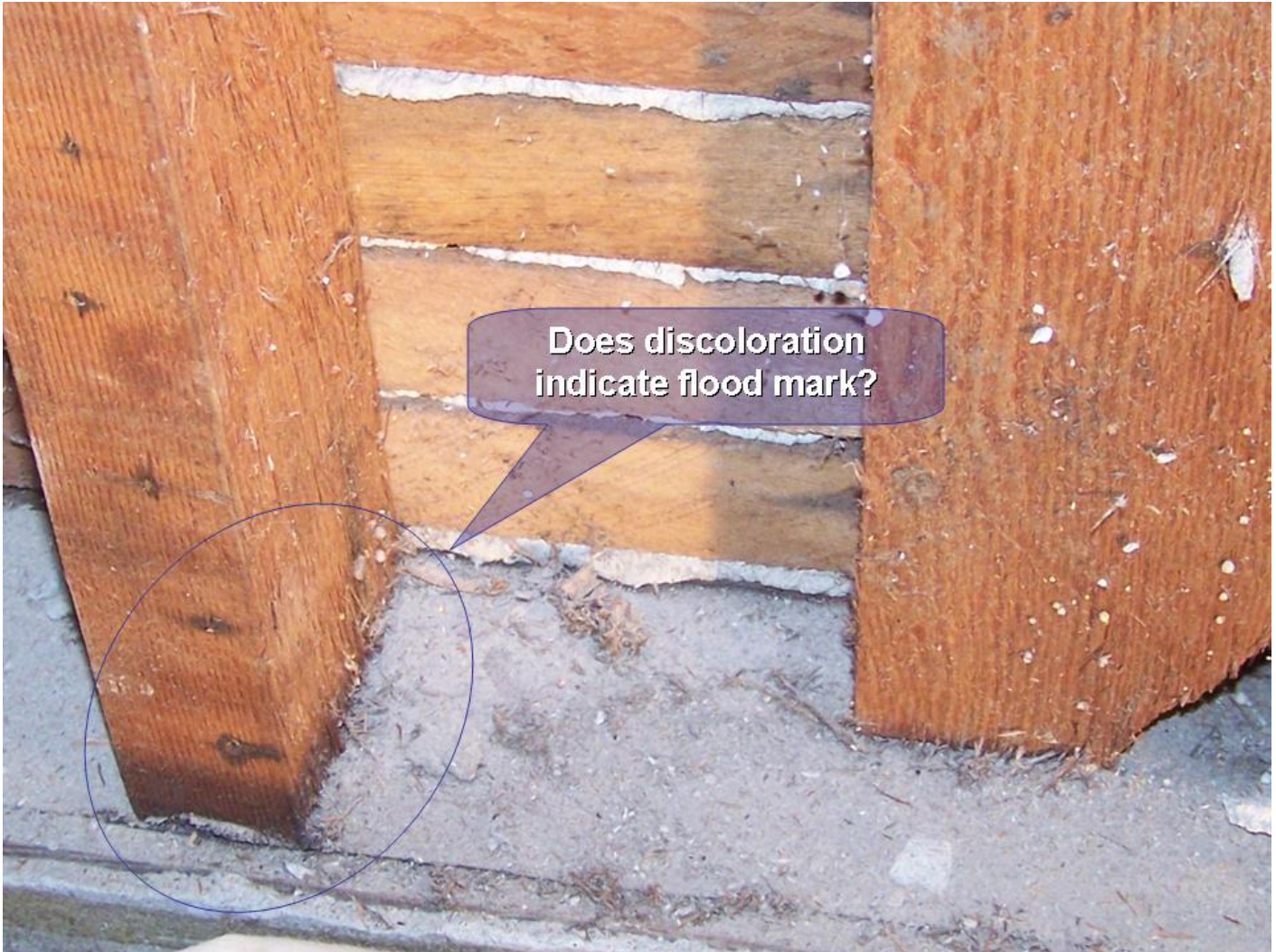
Graphic 8: Close-up of base wall plate.
