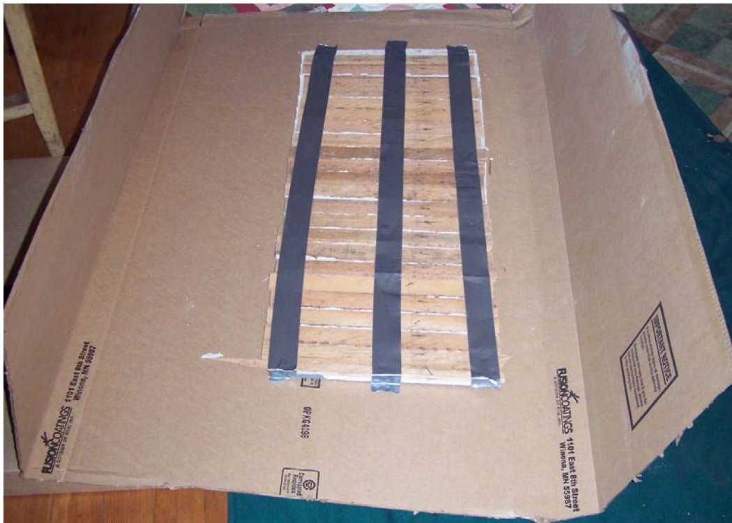
Graphic 5: The lath was reassembled and taped in place to the plaster sections, which came out largely intact.
