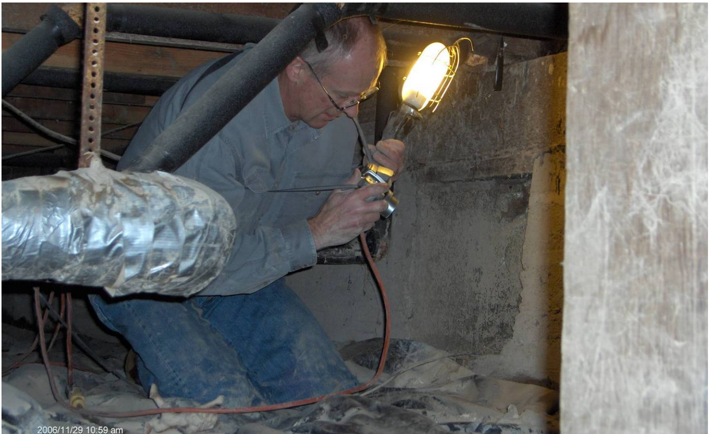
Graphic 14: The original foundation was unaltered. Crawl space observation indicated the house was not elevated.
