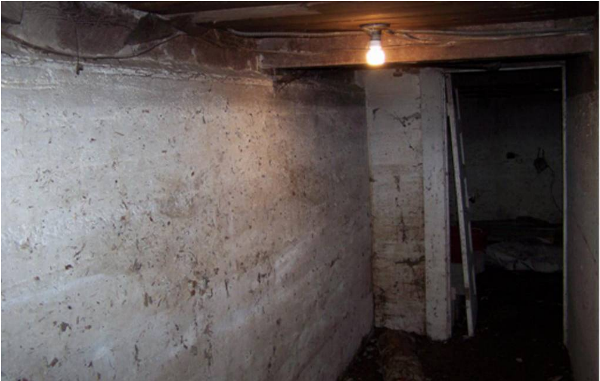
Graphic 13: The original foundation included a basement under approximately a third of the house. Good access enabled easy visual verification that the substructure framing of the house had not been modified or elevated.
