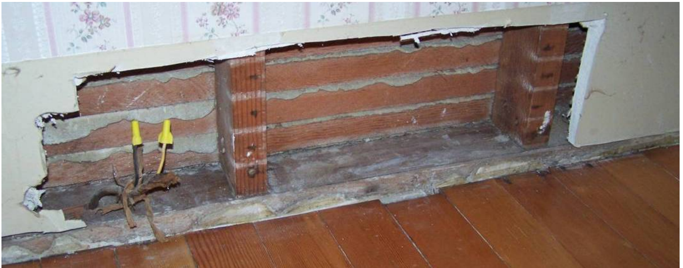
Graphic 11: 2nd cut between the dining room and kitchen, from the dining room side. Lath/plaster had been replaced with gypsum wall board on the dining room side.
