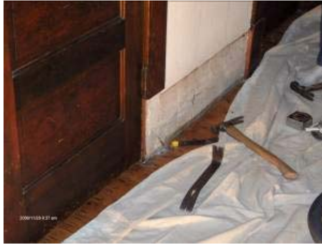
Graphic 4: Photo taken before the first cut with floorboard removed.
