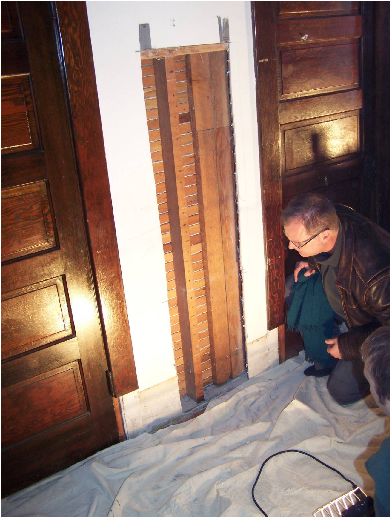
Graphic 10: The first cut was extended to a total of 5'3" in height to observe the interior above the original cut to preclude the possibility that a flood mark existed above the level of the initial cutout.
