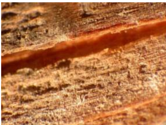
Figure 3. F-3 612 Fairhaven - Locally heavy gray deposits and black biological material on wood surface. Magnification approximately 10X.
