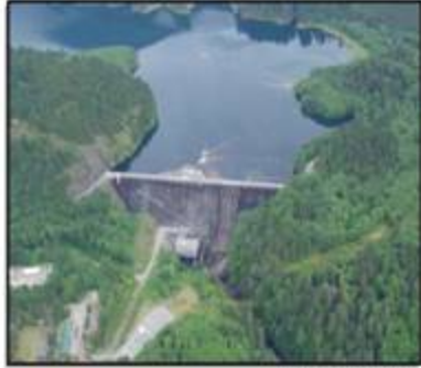
Upper Baker Dam
