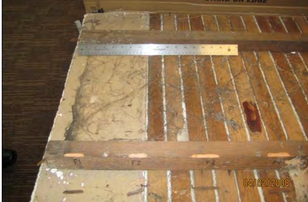
Photo 9. 612 Fairhaven, wall panel removed. Note apparent flood mark to the left of the F3" sample.
