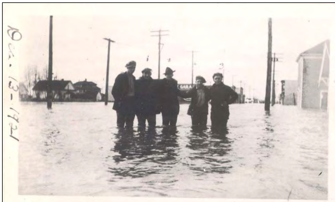
Photo 2. 1921 flood at Fairhaven and Anacortes Street (Figure 27 from Seattle District, Corps of Engineers Revised Flood Insurance Study – Hydraulics May 2008)
