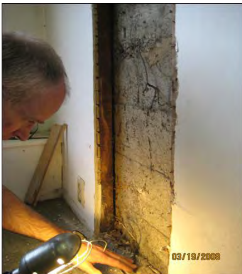
Photo 8. Removal of wall section for forensic investigation. Note bottom lath/plaster has been replaced. Was this due to flooding, or to install electric outlets? Or perhaps both?
