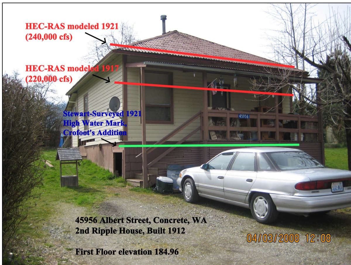
Figure 13. Ripple House #2, parcel #P70748. First floor elevation 184.96. Annotated photo showing with exterior siding removed for inspection of interior wall cavity
