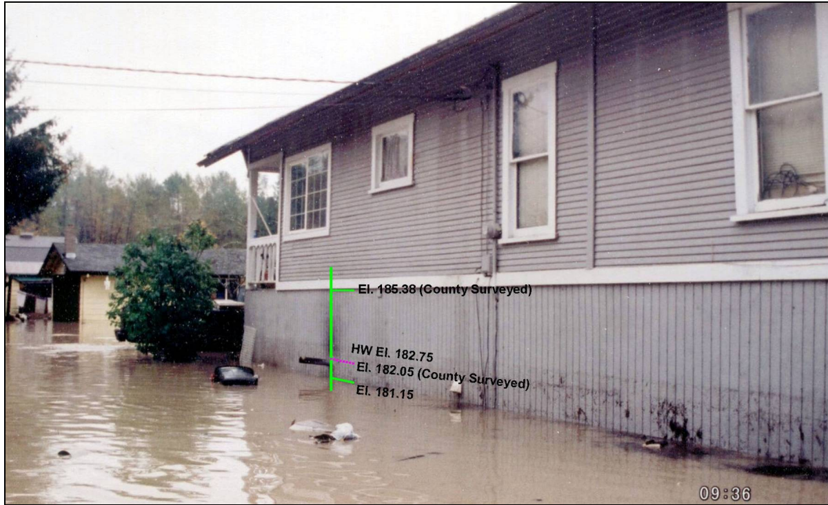
Figure 6. October 2003 Flood – Jenkins House at 7752 South Dillard (RM. 56.18) in Concrete. Photo provided by Allen Jenkins
