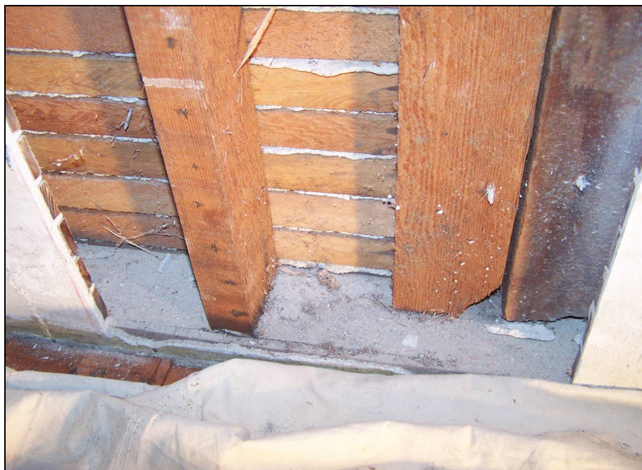
Figure 4. Interior wall cavity, Smith House, 2006.
