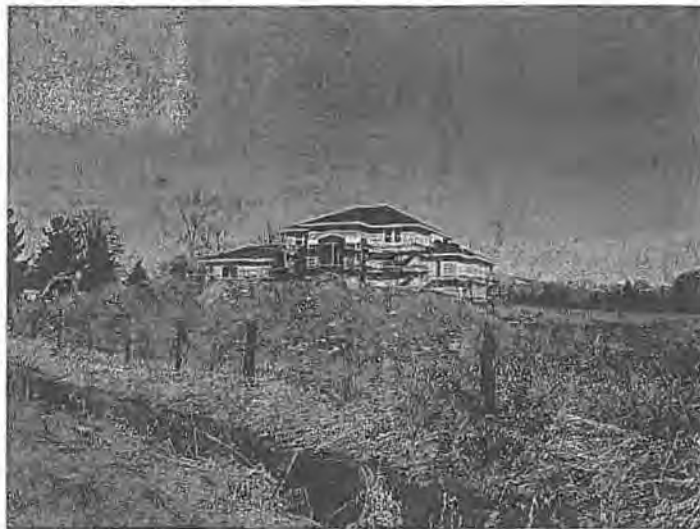
Massive fill being placed in a flow path just upstream and adjacent to Gages Slough in an area where the levees broke in January 1935. See 1/31/35 C.H.
