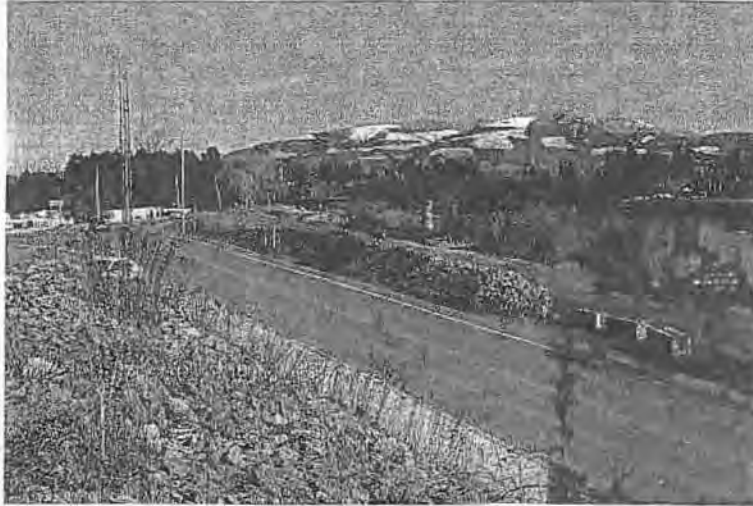
4 feet of fill material placed on the riverward side of the levee in 1990, in the floodway just 6 years after the adoption of the local flood ordinance.
