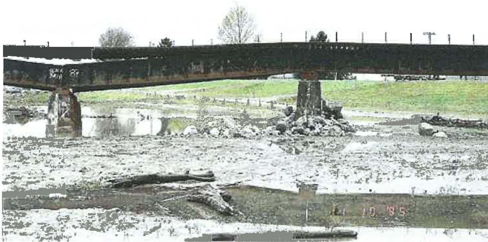
BNSF Skagit River Bridge, November, 1995
