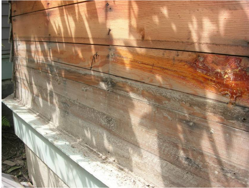
Figure 9. Smith House, Opening No. 4. Water line at approximately same elevation as finish floor line behind lap siding.
