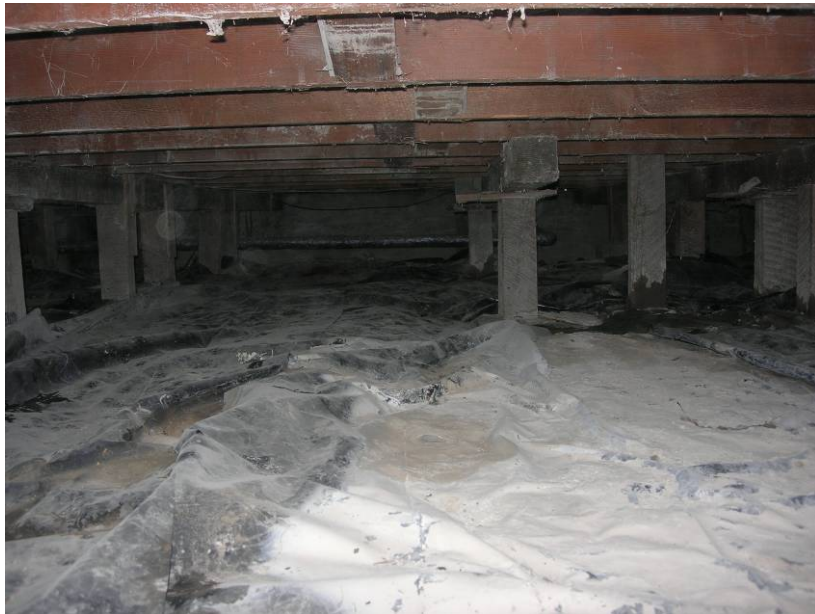
Figure 6. Smith House crawlspace.
