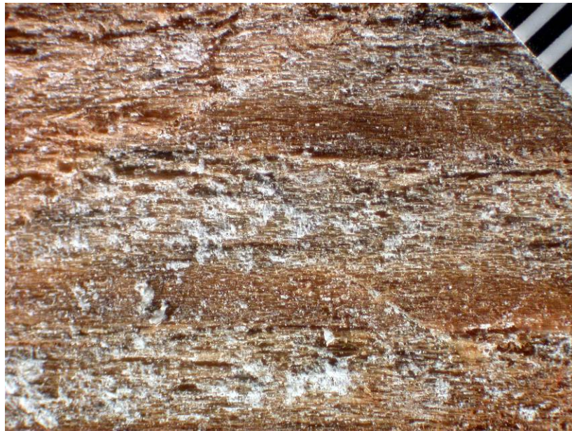
Figure 42. Closer view of deposits on lath. Millimeter scale.
