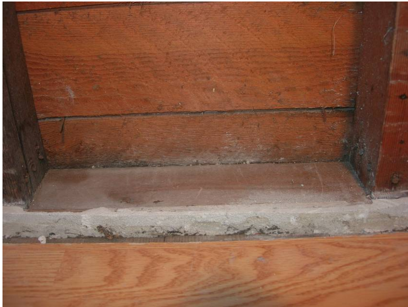
Figure 8. Close-up view of Opening No. 2. No water lines present.
