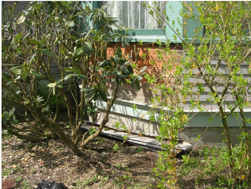
Figure 4. Smith House, Opening No. 4. North exterior wall behind siding.
