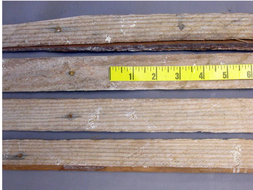
Figure 41. Opening No. 2, front surface of lath slats.
