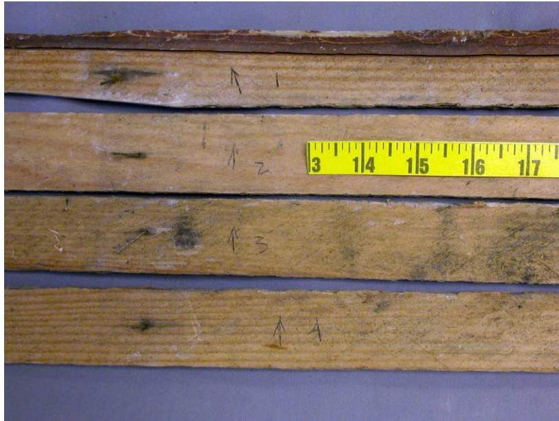
Figure 40. Opening No. 2 East Exterior Wall, back surface.
