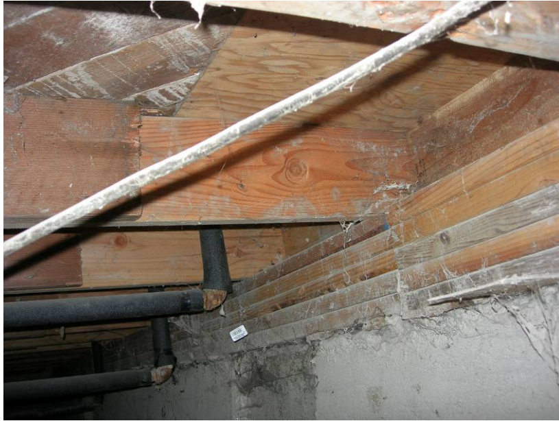
Figure 7. Repairs at south end of Smith House foundation.
