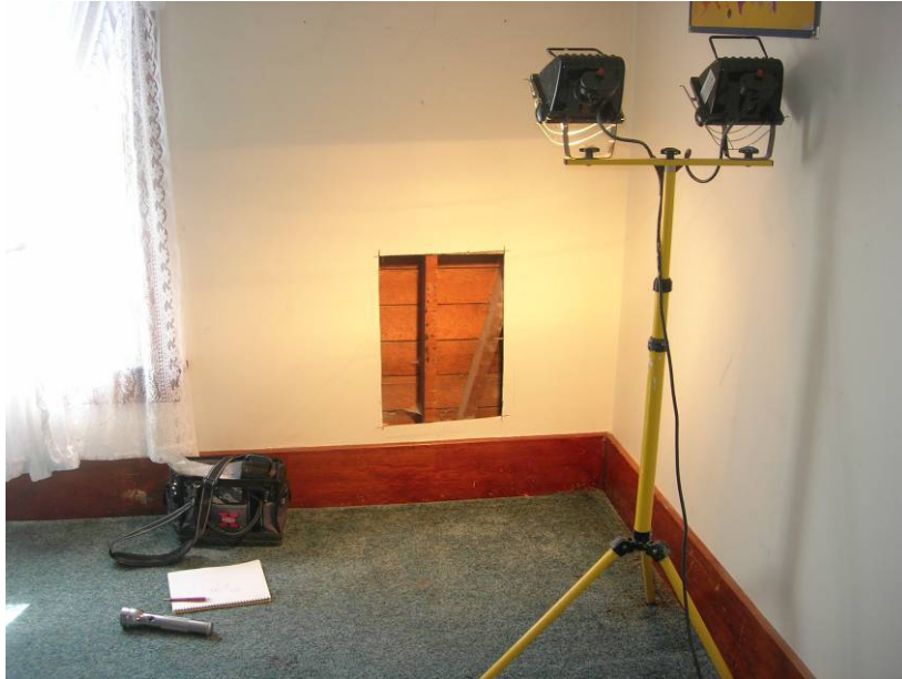
Figure 1. Smith House, Opening No. 1. Upstairs bedroom, north exterior wall.
