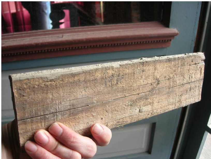
Figure 10. Grey deposits on top of sheathing boards at Slipper House interior wall opening.
