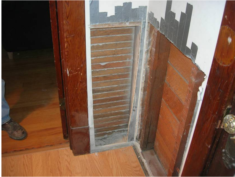
Figure 3. Smith House, Opening No. 3. Opening at south side of interior wall adjacent to Opening No. 2.
