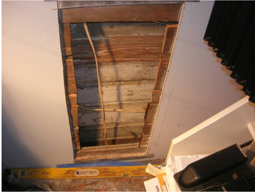
Figure 5. Slipper House, Opening No. 5. Opening at interior office wall.
