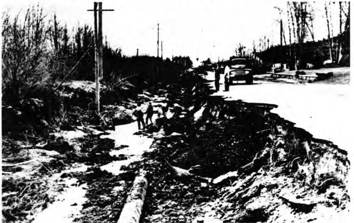
Fig. A-2. Erosion damage to Burlington water main and State Highway 1 between Burlington and Sedro Woolley caused by the February 1951 Flood. (Soil Conservation Service Photo)
