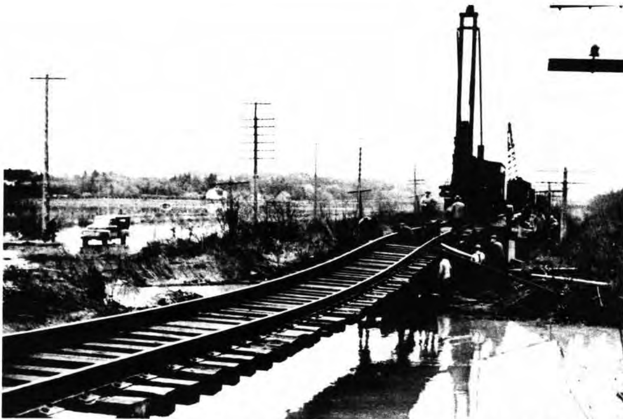
Fig. A-3. Maintenance crew preparing to rebuild a section of the Great Northern mainline south of Conway, washed out during the November 1949 Flood. (Soil Conservation Service Photo)
