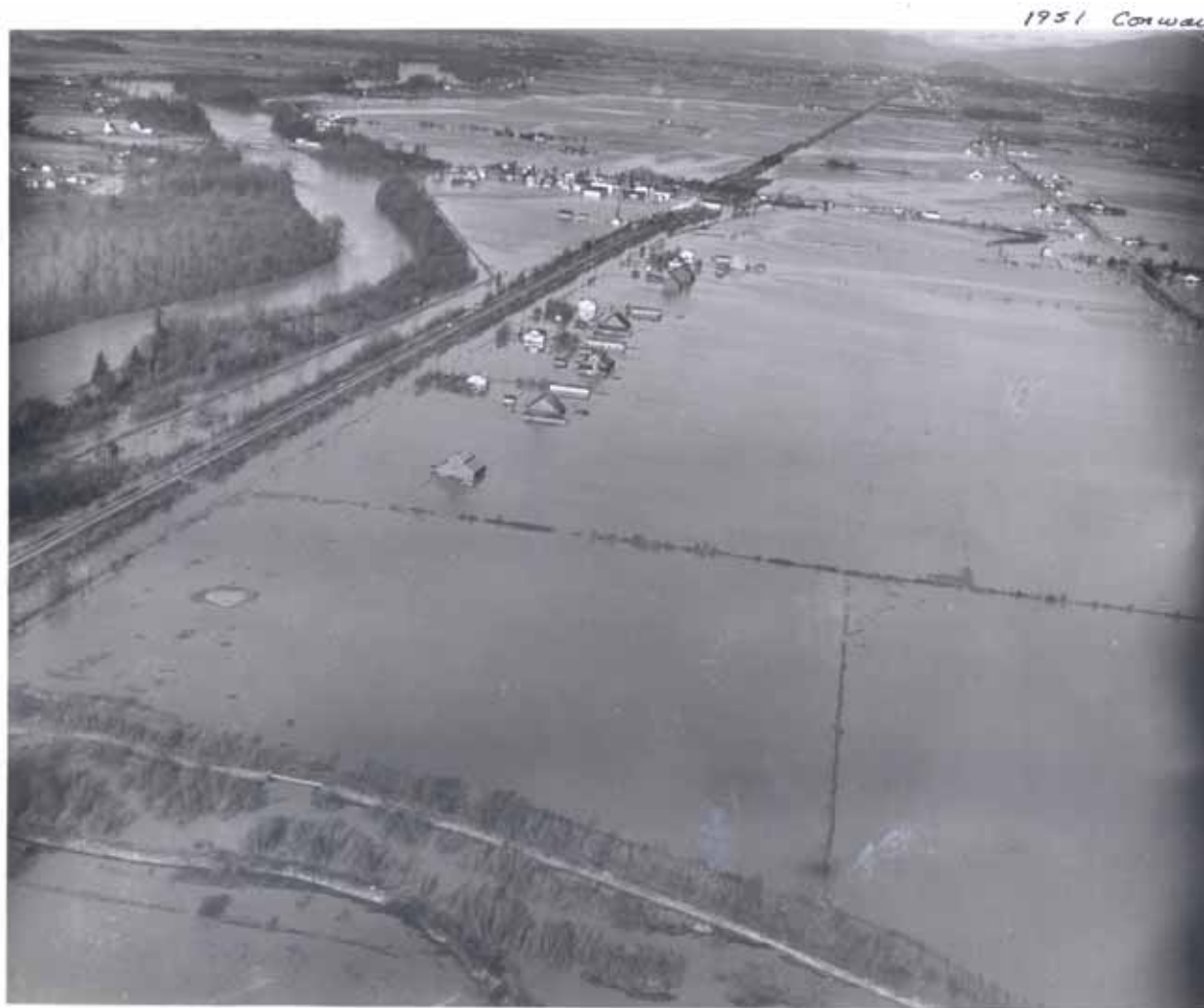
Figure 30 – Conway Area in February 1951 Flood
