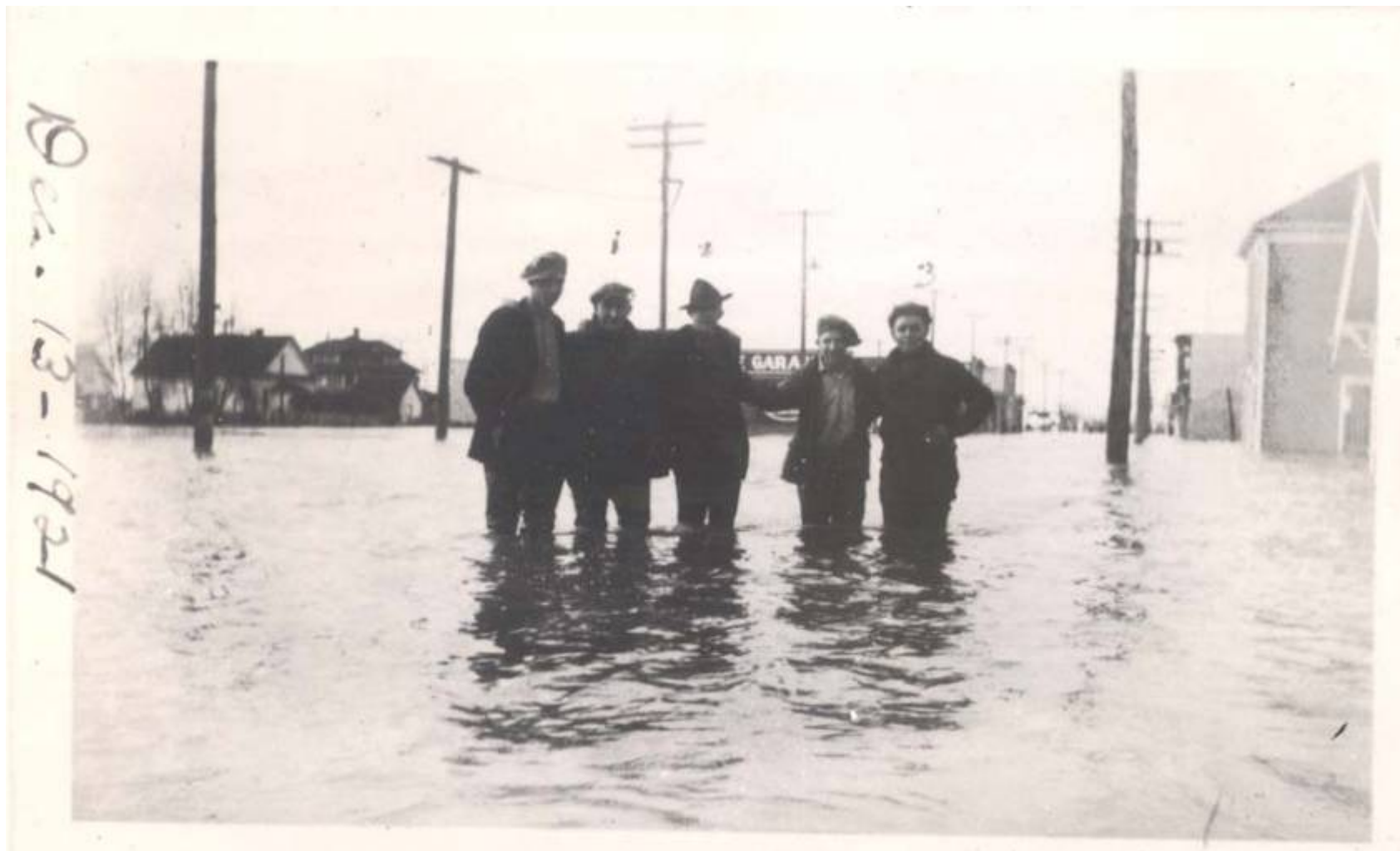
Figure 27 – December 1921 Flood at Fairhaven and Anacortes Streets
