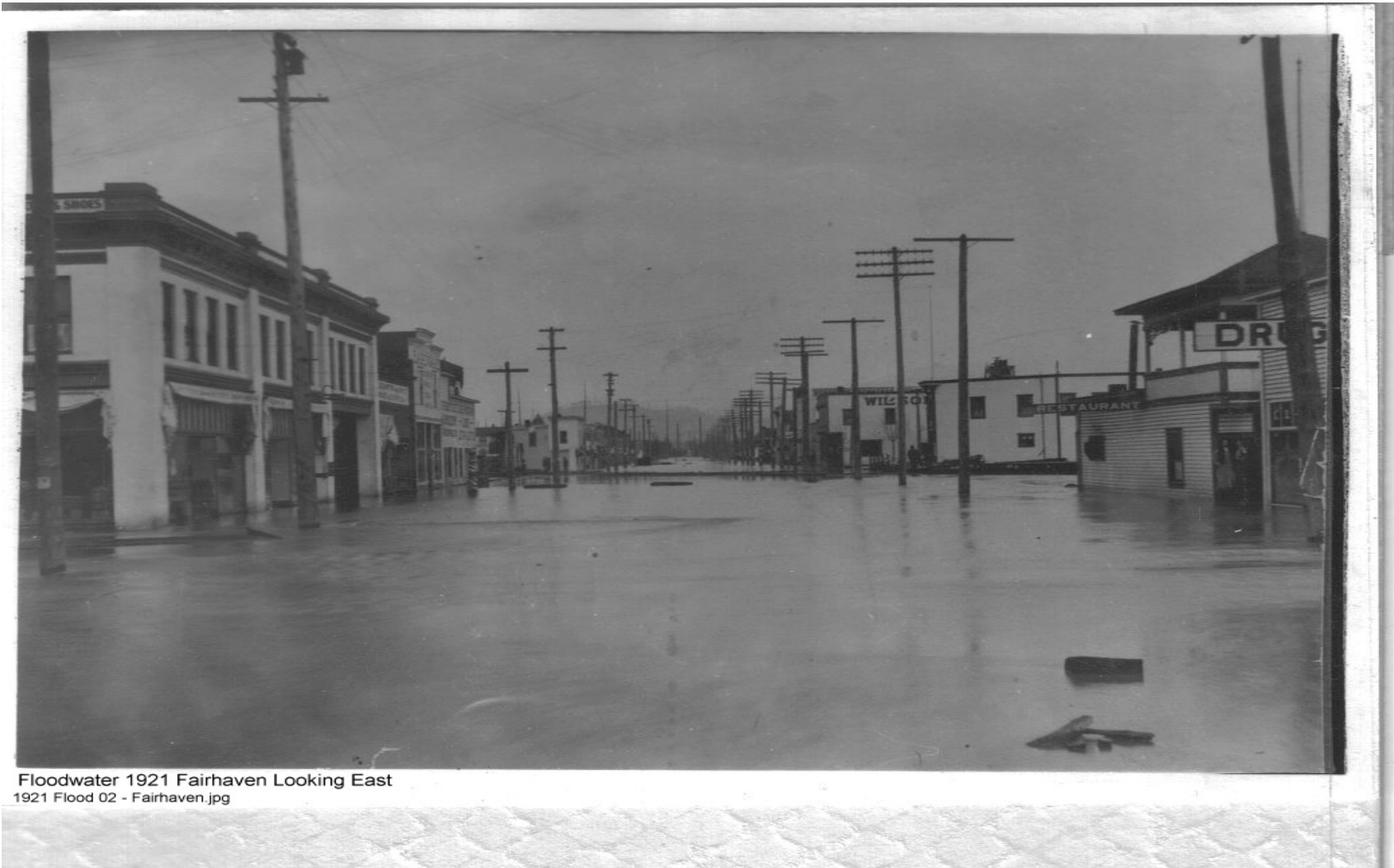
Figure 28 – December 1921 Flood at Fairhaven Street
