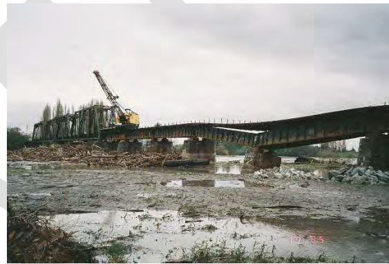
Figure 4a and 4b: Debris accumulation on the BNSF Bridge during 1995 flood event looking upstream.
