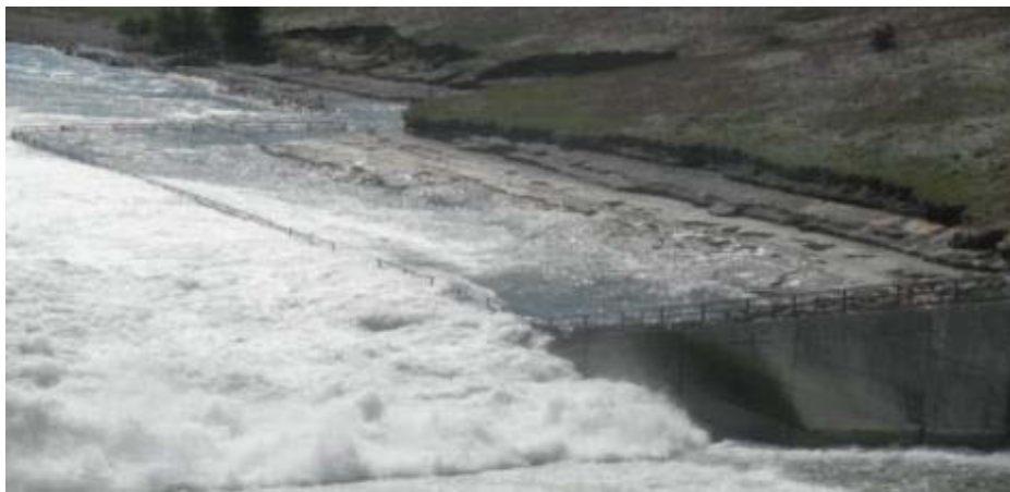
Figure 88. Dams damage/erosion: Big Bend Erosion on earthen walls of the project's spillway in South Dakota
