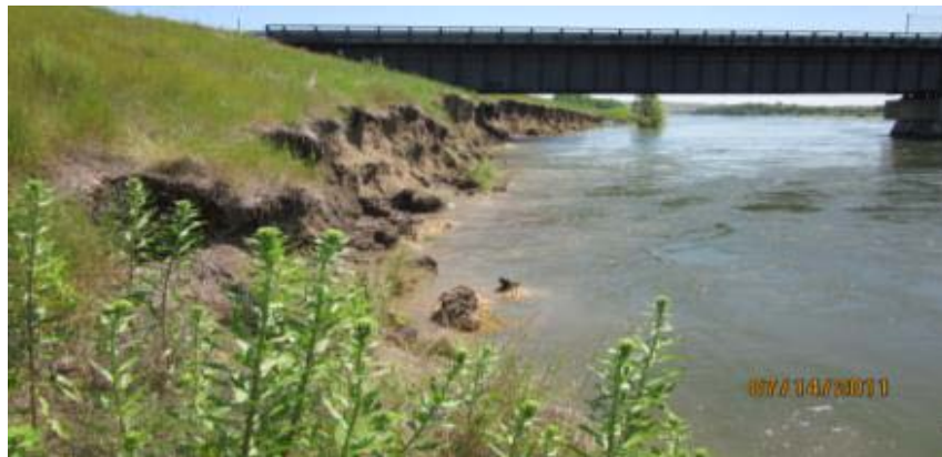
Figure 84. Dams damage/erosion: Oahe - Outlet works bridge scour at abutment at Oahe, South Dakota
