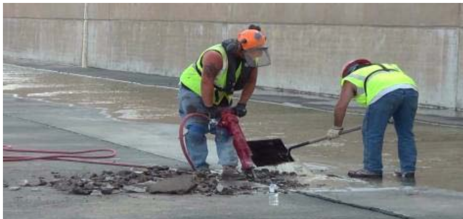
Figure 72. Dams damage/erosion: Garrison - Typical concrete repair from flood in North Dakota. Additional spall repairs needed at most dams.
