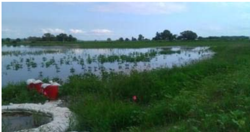
Figure 103. Levee seepage/sandboils: Typical landside seepage and sandboils at L611-614 near Council Bluffs, Iowa
