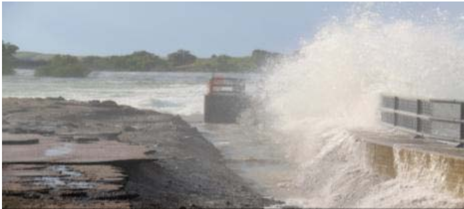
Figure 81. Dams damage/erosion: Oahe
