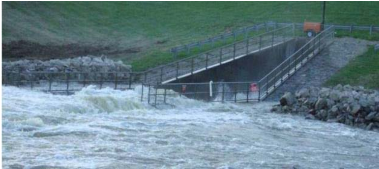
Figure 14. Rathbun Stilling Basin Overtopping at 3,000 cfs
