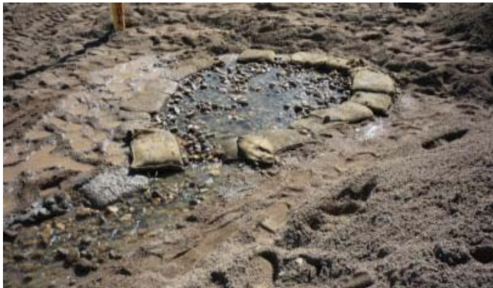
Figure 67. Levee boils: Williston - Additional relief wells needed at Williston Levee in North Dakota
