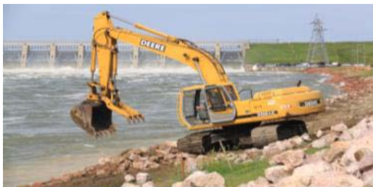
Figure 99. Dams damage/erosion: Gavins Point - Erosion on earthen walls of the project's spillway in South Dakota (under repair)
