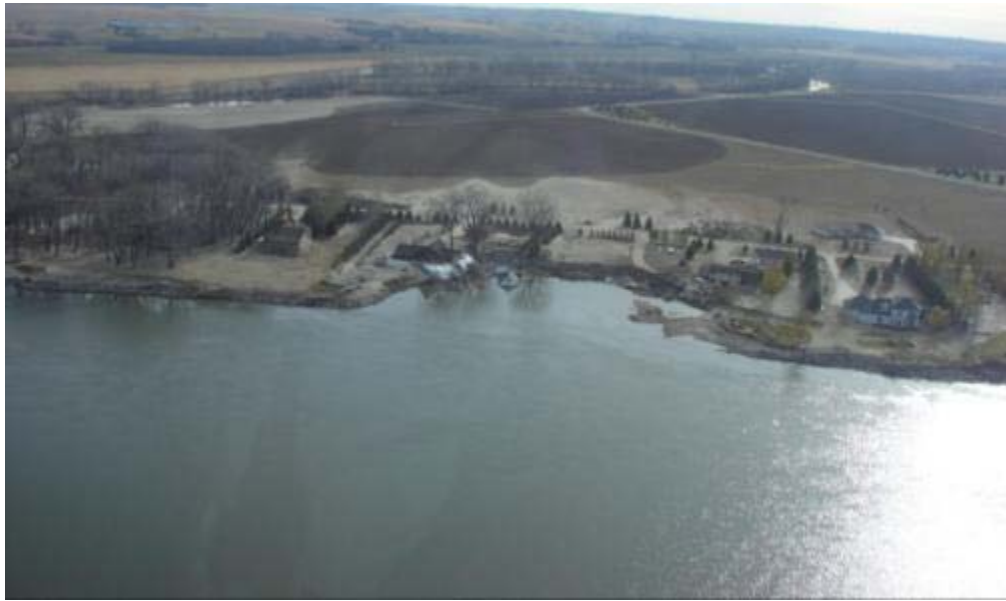
Figure 76. Erosion: Hogue Island, Section 33 Project - Erosion along the Section 33 Project at Hogue Island, North Dakota
