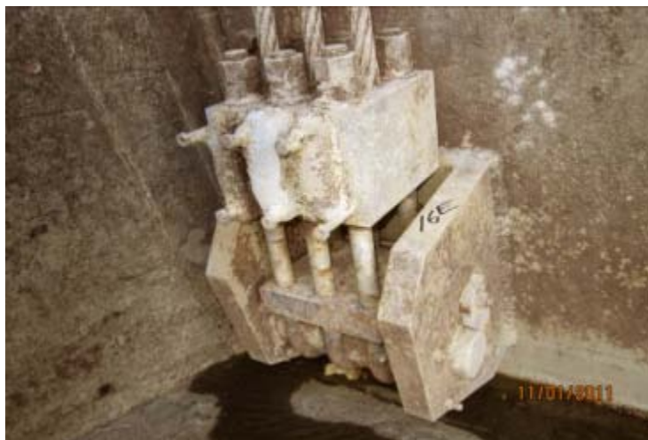
Figure 94. Dams damage/erosion: Fort Randall - spillway gate wire rope hoist linkage corrosion
