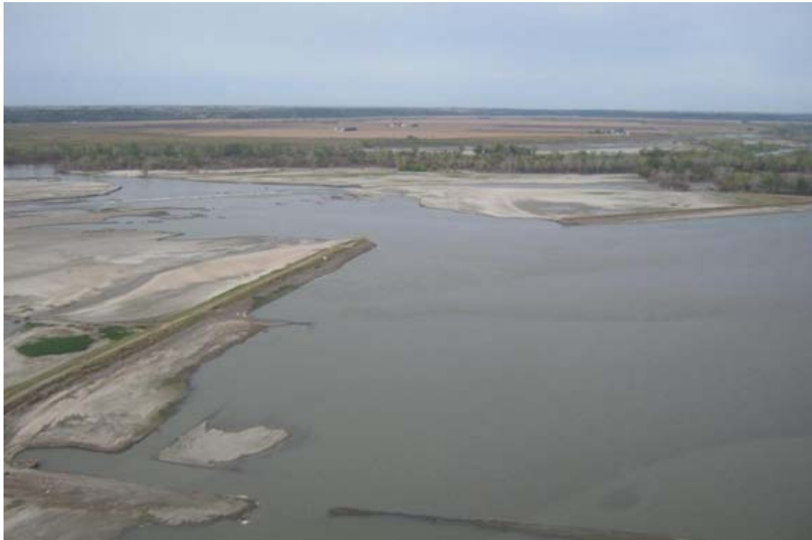
Figure 109. Levee breach: Lower breach at L575
