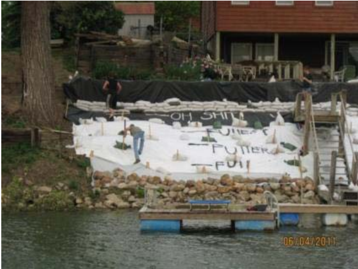
Figure 36. Kensler's Bend Project at Dakota Dunes along Left Bank River Mile 737
