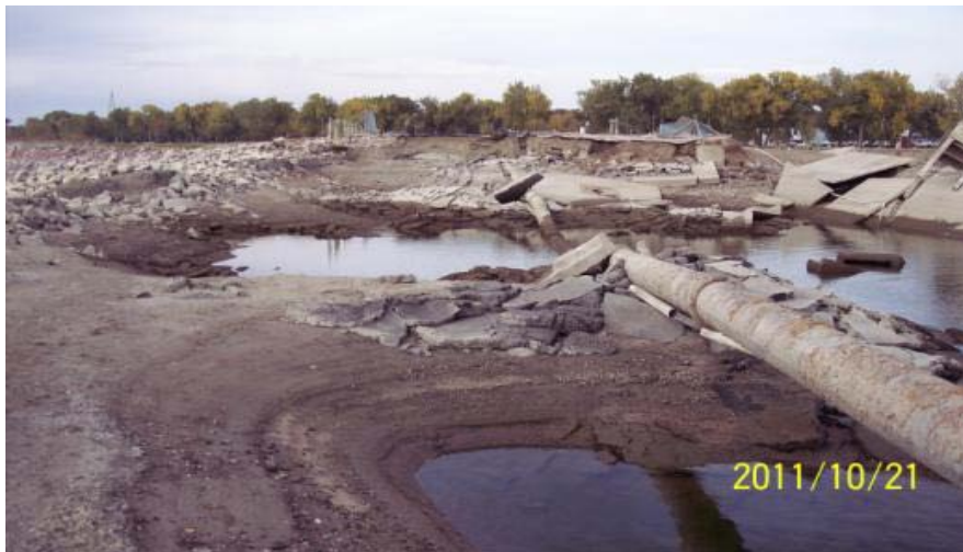
Figure 85. Damage/erosion: LaFramboise Island Causeway - City of Pierre waterlines damaged at LaFramboise Island Causeway (Corps) in Pierre, South Dakota
