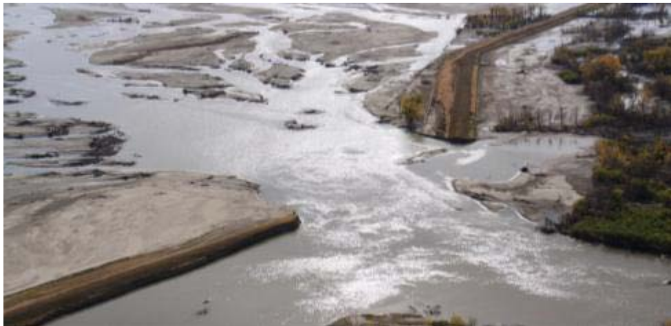
Figure 107. Levee breach: Middle breach at L575
