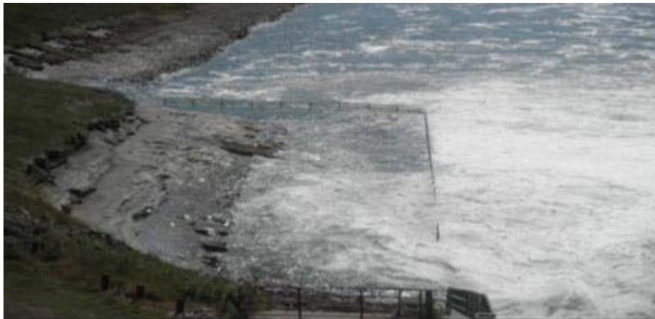
Figure 87. Dams damage/erosion: Big Bend Erosion on earthen walls of the project's spillway in South Dakota
