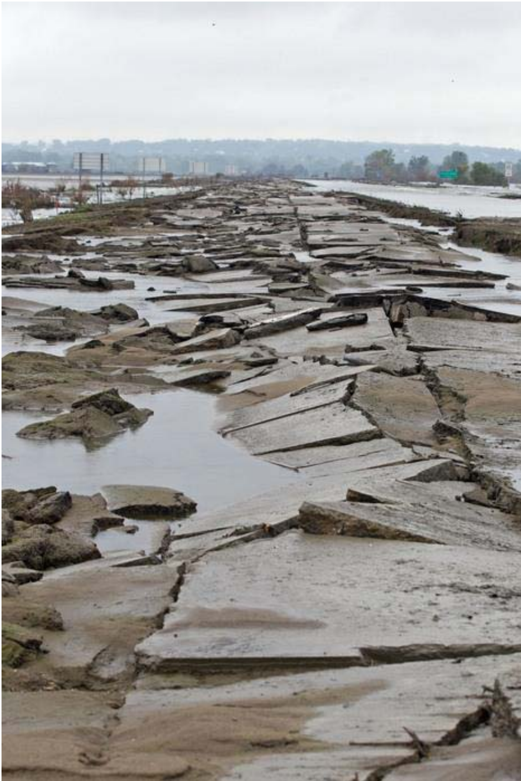
Figure 10. Omaha World Herald Photo: The flood-damaged eastbound lane of Interstate I-680, looking west toward the Mormon Bridge from the overpass over I-29. Receding water from the flooded Missouri River revealed flood damage north of Council Bluffs.
