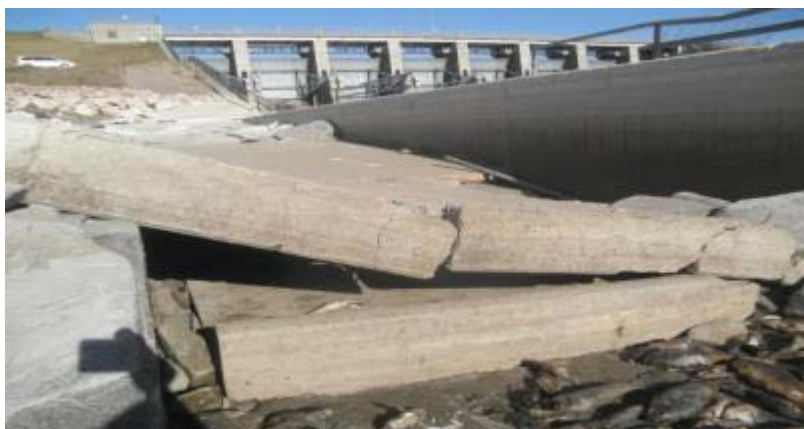
Figure 91. Dams damage/erosion: Big Bend – Project's spillway overtopping damage in South Dakota currently under repair
