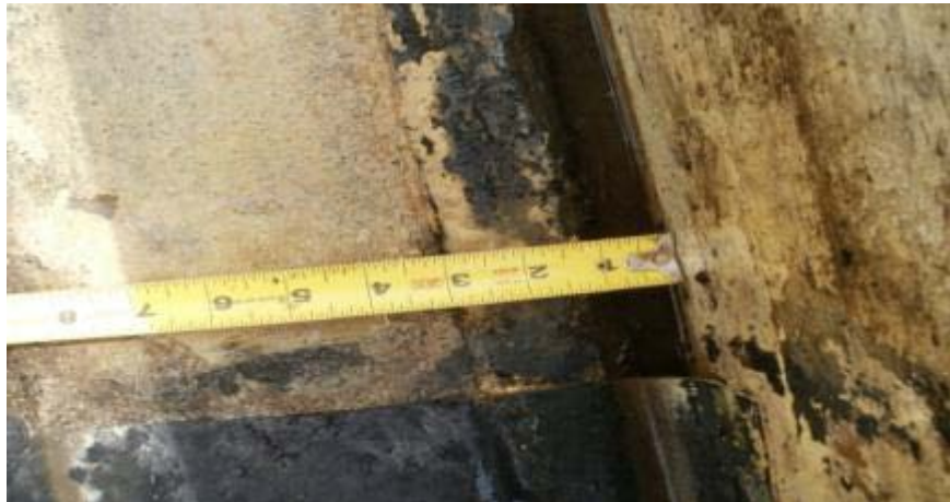
Figure 73. Dams damage/erosion: Garrison - Joint separation and seal repairs required at Garrison Dam in North Dakota
