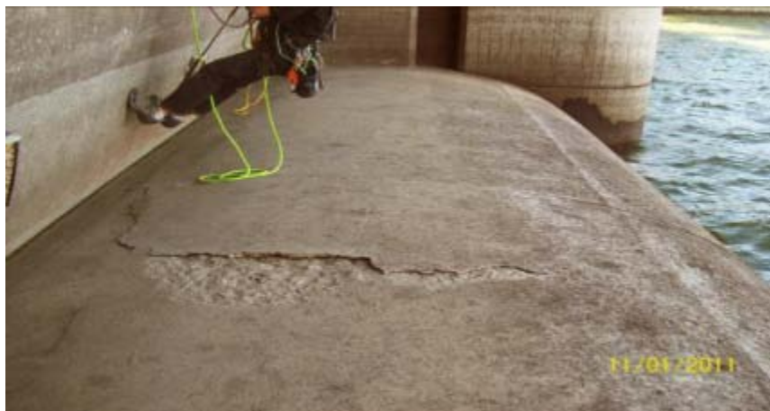
Figure 93. Dams damage/erosions: Fort Randall - Spillway weir spalling
