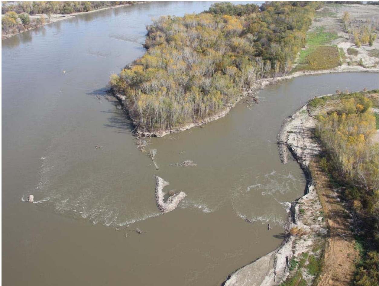
Figure 27. Upper Kansas Bend SWH Chute Inlet at River Mile 546 (facing downstream) - 2011 Post Flood. Flood Erosion Flanked the Stone Protection at the "V" Structure Along the Downstream Bankline
