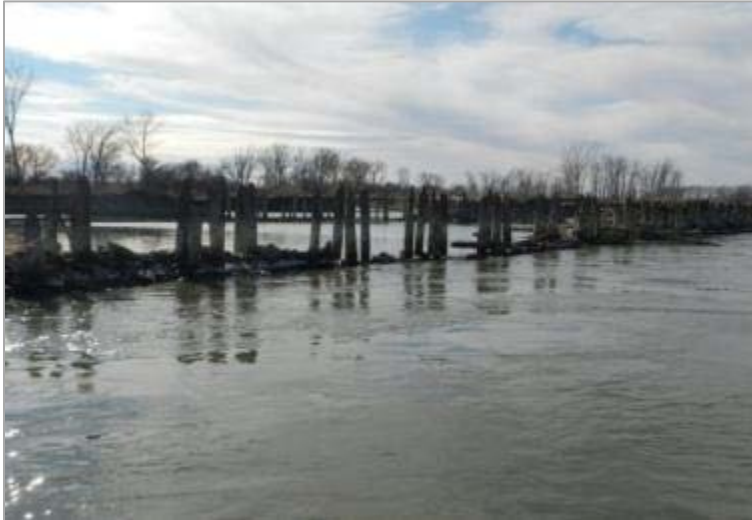
Figure 30. Revetment Near River Mile 679.8
