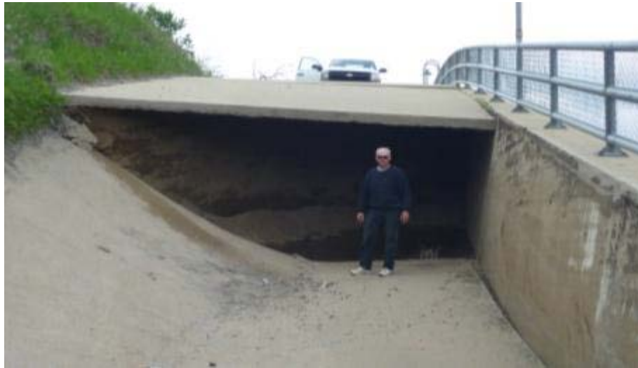
Figure 95. Dams damage/erosion: Fort Randall - Spillway wingwall backfill erosion (currently under repair) at Fort Randall in South Dakota
