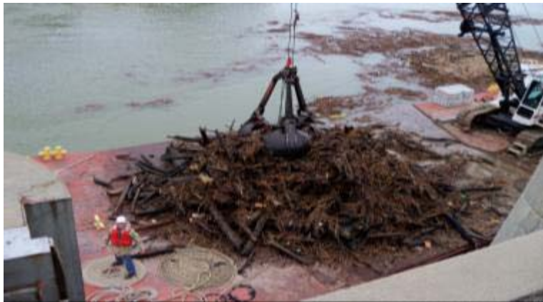
Figure 98. Dams damage/erosion: Gavins Point - Excess debris led to clogging of water intake at Hydropower Plant (under repair) in South Dakota
