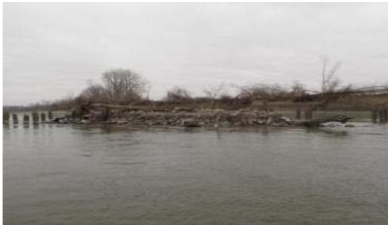
Figure 33. Flanked Dike at River Mile 322.4 on Right Bank.
