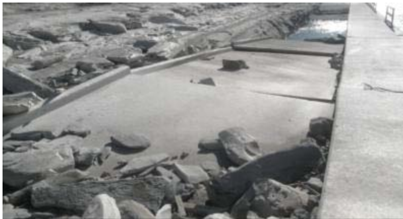
Figure 90. Dams damage/erosion: Big Bend – Project's spillway overtopping damage in South Dakota currently under repair
