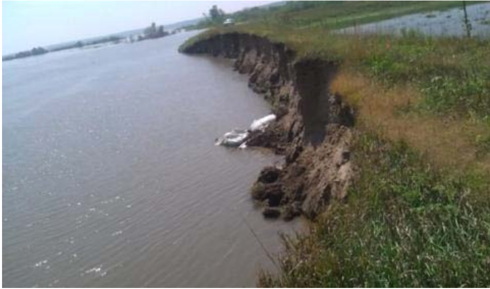
Figure 113. Levee scouring/erosion: L536 - Levee erosion – more than 50 percent of the embankment is missing – at MR Levee L536
