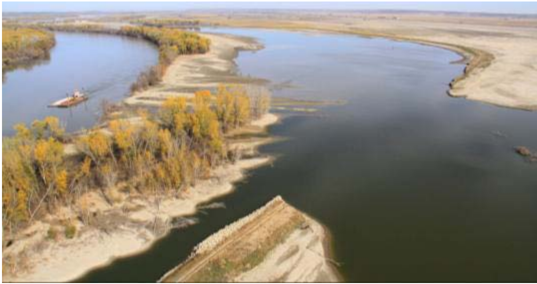
Figure 104. Levee breach: Upper breach at L575
