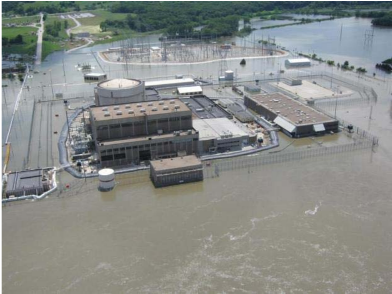
Figure 9. Fort Calhoun Nuclear Station (June 25, 2011)
