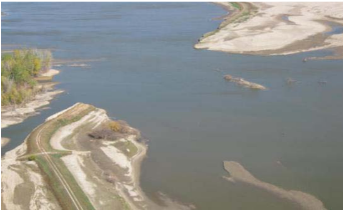
Figure 105. Levee breach: Upper breach at L575
