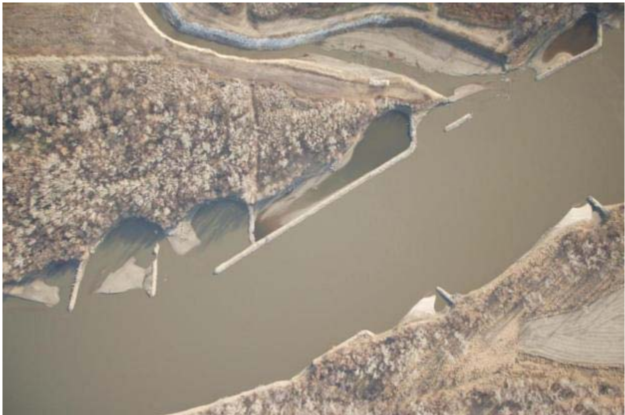
Figure 26. Upper Kansas Bend SWH Chute Inlet at River Miler 546 - Pre Flood 2005. Downstream Flow to Left
