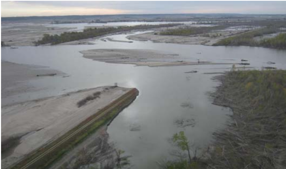
Figure 111. Levee breach: Upper breach at L550
