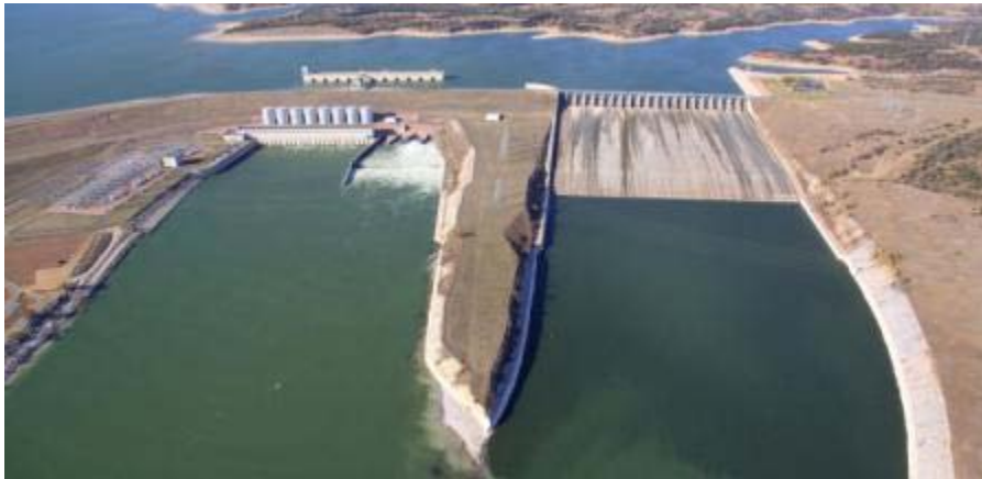
Figure 92. Dams damage/erosion: Fort Randall - Sloughing on earthen walls of the project's spillway and regulating tunnels in South Dakota
