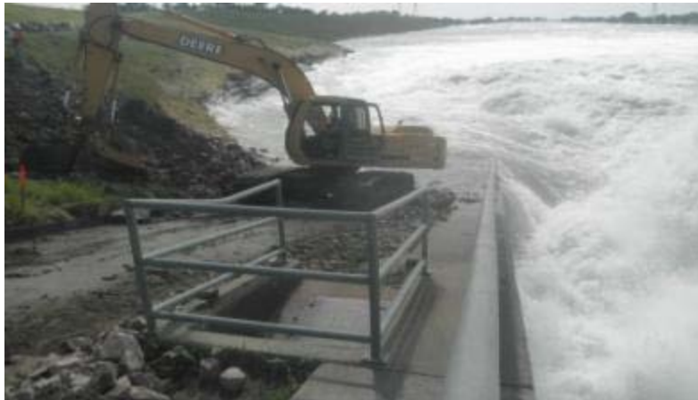
Figure 89. Dams damage/erosion: Big Bend - Project's spillway in South Dakota being overtopped during flood
