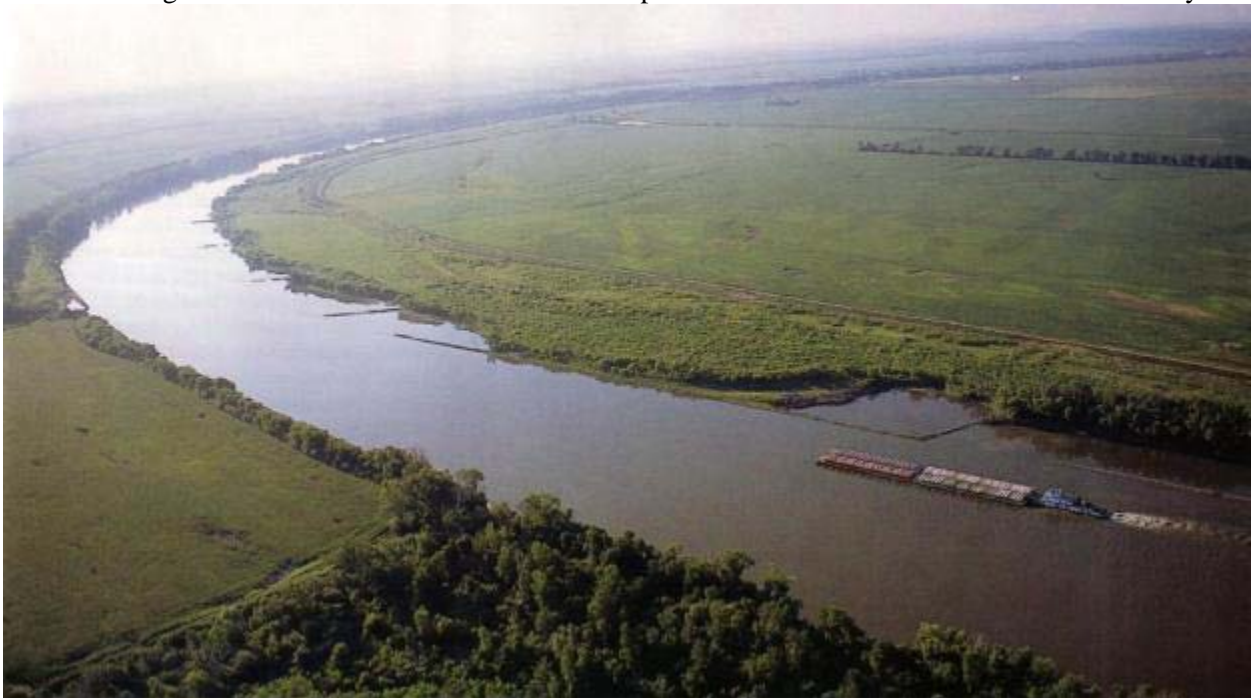
Figure 24. BSNP Channel with Private Levee System along Right Bank near Indian Cave State Park, Nebraska River Mile 517 Prior to 2011 flood.
