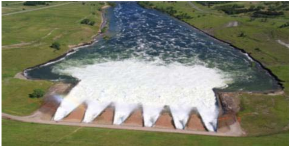
Figure 80. Dams damage/erosion: Oahe - Erosion along the earthen walls extending from Oahe's stilling basin outside Fort Pierre, South Dakota
