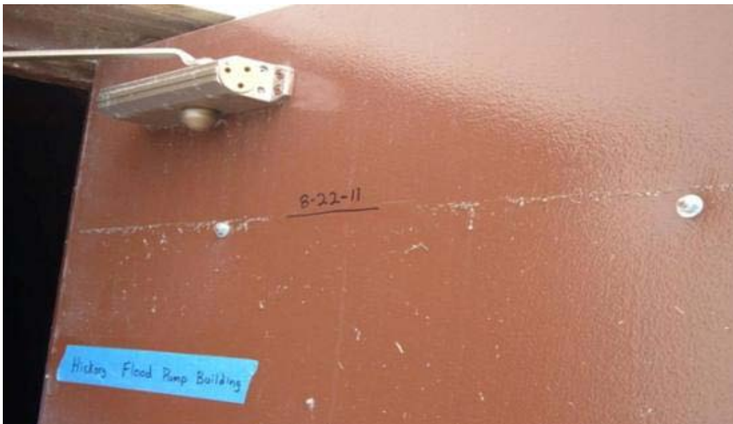
Figure 101. Flood protection project damage: Hickory Street Pump Station - High water mark on interior side of an exterior door at a flood protection project in Omaha, Nebraska
