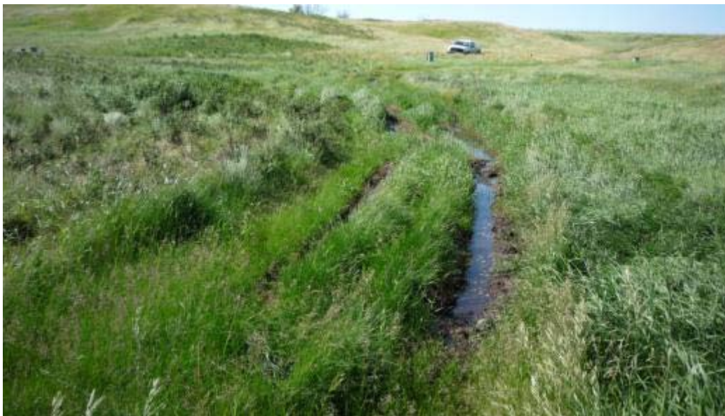
Figure 77. Dams damage/erosion: Pipestem Dam - Downstream right abutment seepage area at Pipestem Dam in South Dakota
