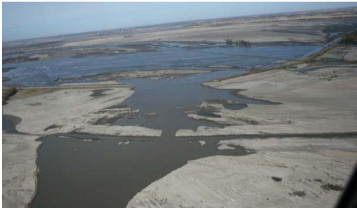
Figure 110. Levee breach: Lower breach at L575
