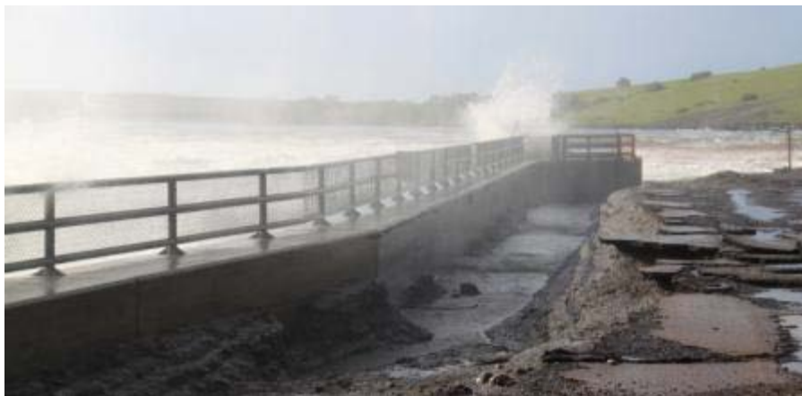
Figure 82. Dams damage/erosion: Oahe - Erosion at flood tunnel outlet for Oahe outside Fort Pierre, South Dakota (under repair)
