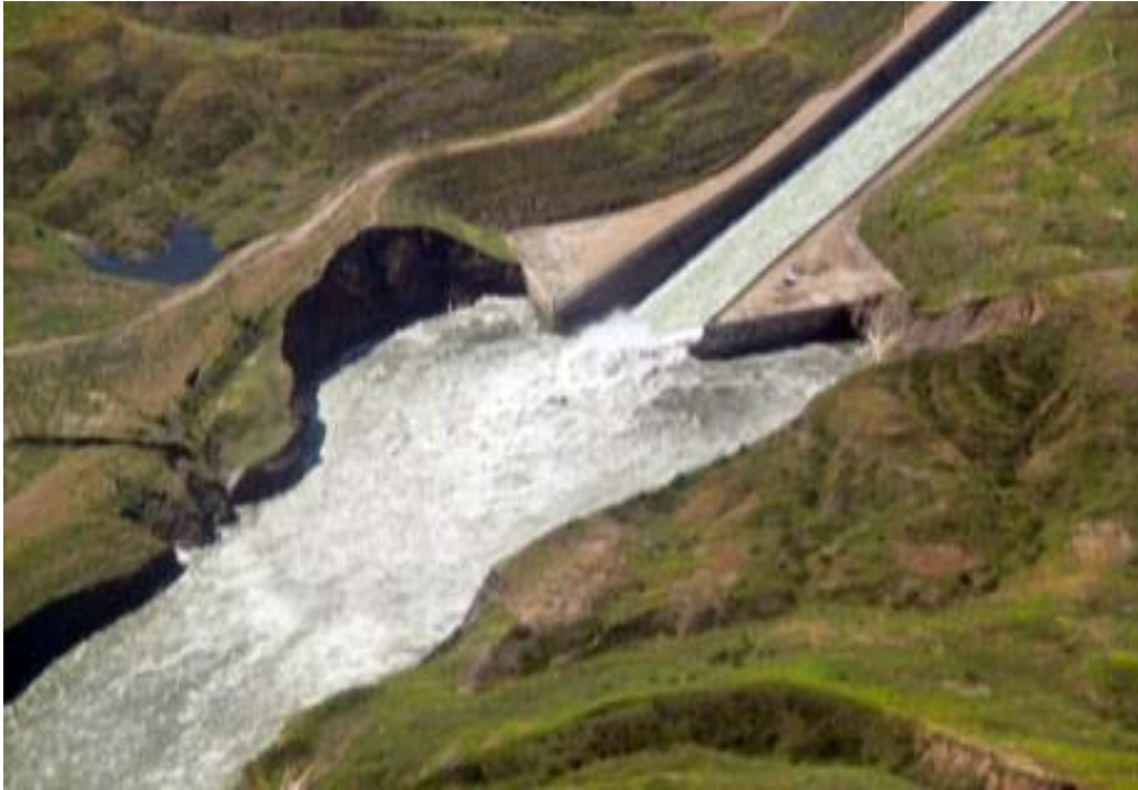
Figure 65. Dams damage/erosion: Fort Peck - Erosion along the spillway plunge pool extending from Fort Peck's spillway in Fort Peck, Montana
