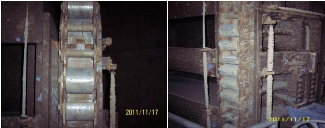
Figure 83. Dams damage/erosion: Oahe - Flood control tunnel gate roller chain failure at Oahe outside Fort Pierre, South Dakota
