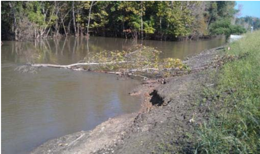
Figure 102. Levee scouring/erosion: Typical riverside erosion and vegetation loss at L611-614 near Council Bluffs, Iowa
