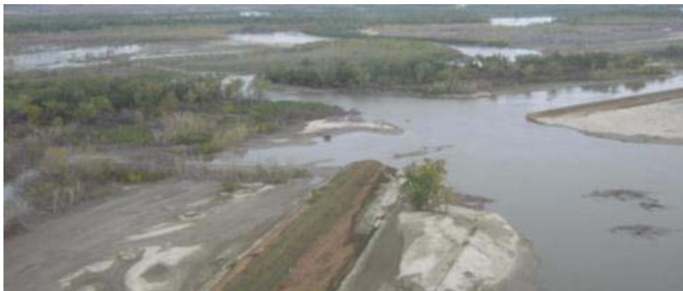
Figure 108. Levee breach: Middle breach at L575
