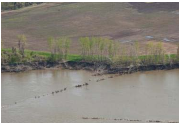
Figure 34. Dike and Revetment Damage at River Mile 250.5
