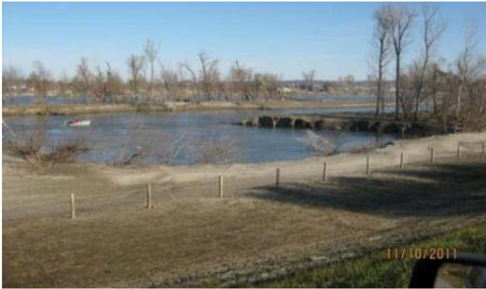
Figure 100. Levee scouring/erosion: Scour hole between Council Bend chute and MR Levee L624-627 toe in Council Bluffs, Iowa
