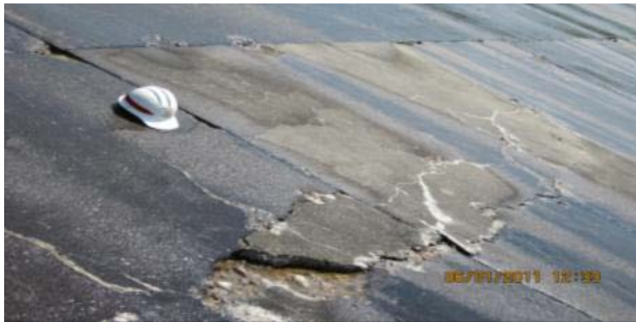
Figure 71. Garrison Spillway damage/erosion:
