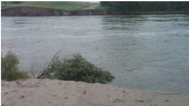
Figure 74. Dams damage/erosion: Garrison - Erosion along the earthen walls extending from Garrison Dam's spillway apron in North Dakota
