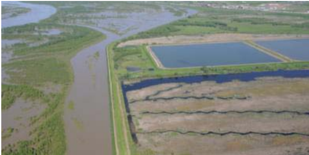
Figure 66. Levee seepage: Williston - Landside seepage, relief wells needed at Williston Levee, North Dakota
