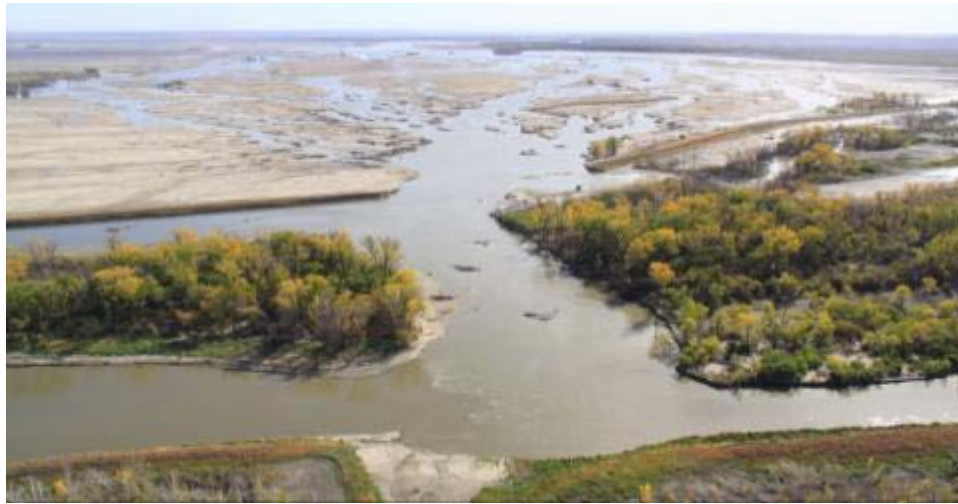
Figure 106. Levee breach: Middle breach at L575
