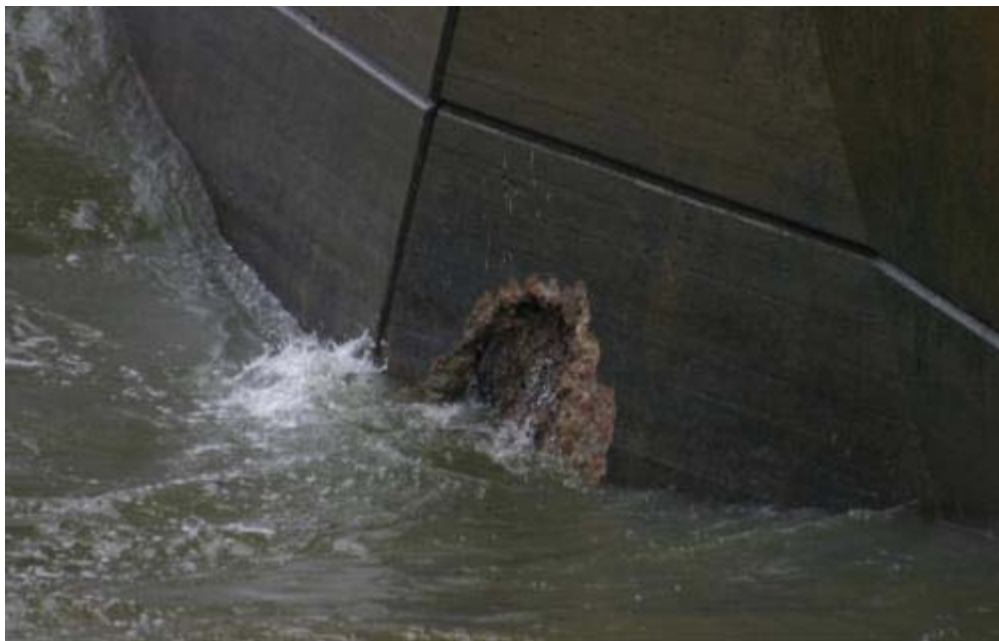
Figure 96. Dams damage/erosion: Fort Randall - Downstream spillway wingwall concrete spall at Fort Randall, South Dakota
