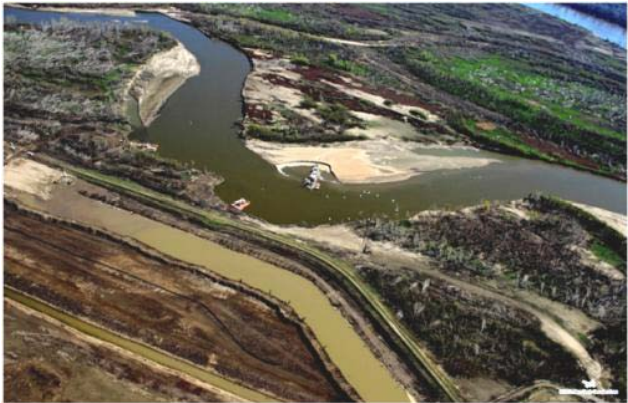
Figure 28. Upper Hamburg Bend Levee Toe Scour Repair Area
