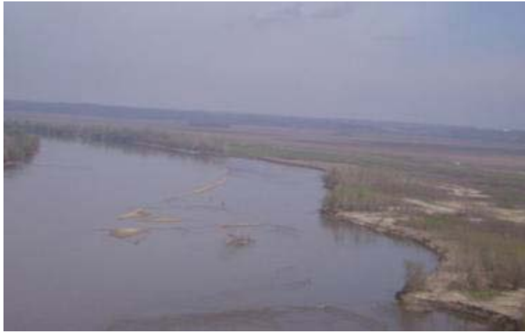
Figure 32. Wolf Creek Bend Revetment Chute Erosion
