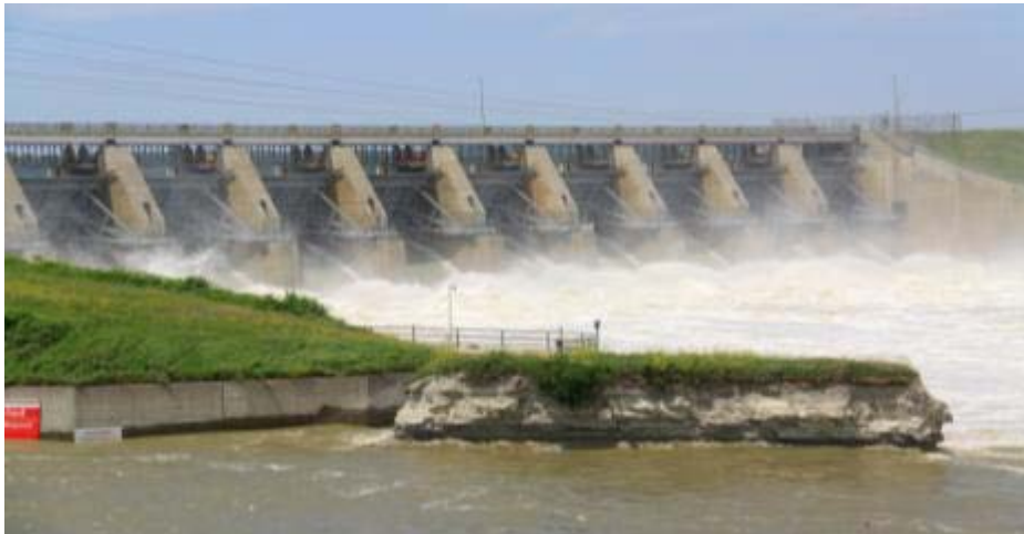
Figure 97. Dams damage/erosion: Gavins Point - Erosion on earthen walls of the project's spillway in South Dakota
