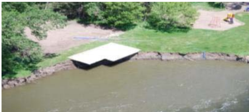
Figure 75. Dams damage/erosion: Garrison - Downstream camp erosion at Garrison Dam in North Dakota
