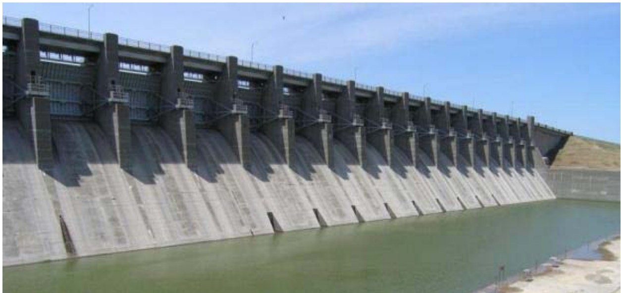
Figure 15. Harlan County Spillway and Stilling Basin
