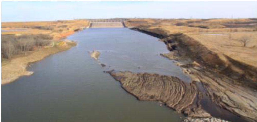
Figure 70. Dams damage/erosion: Garrison - Erosion along the earthen walls extending from Garrison Dam's spillway apron in North Dakota
