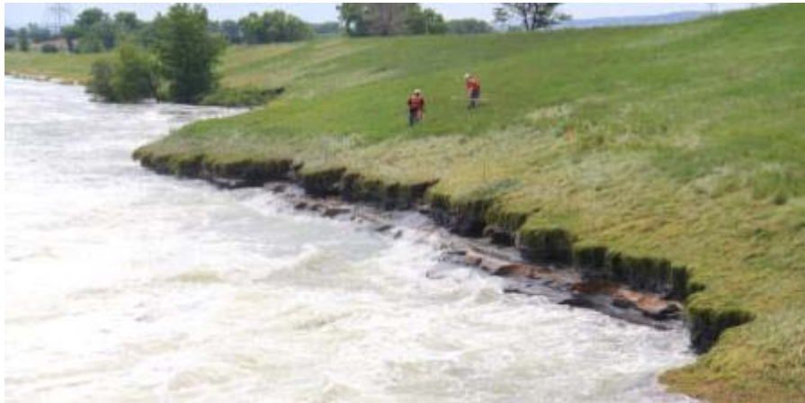
Figure 86. Dams damage/erosion: Big Bend Erosion on earthen walls of the project's spillway in South Dakota
