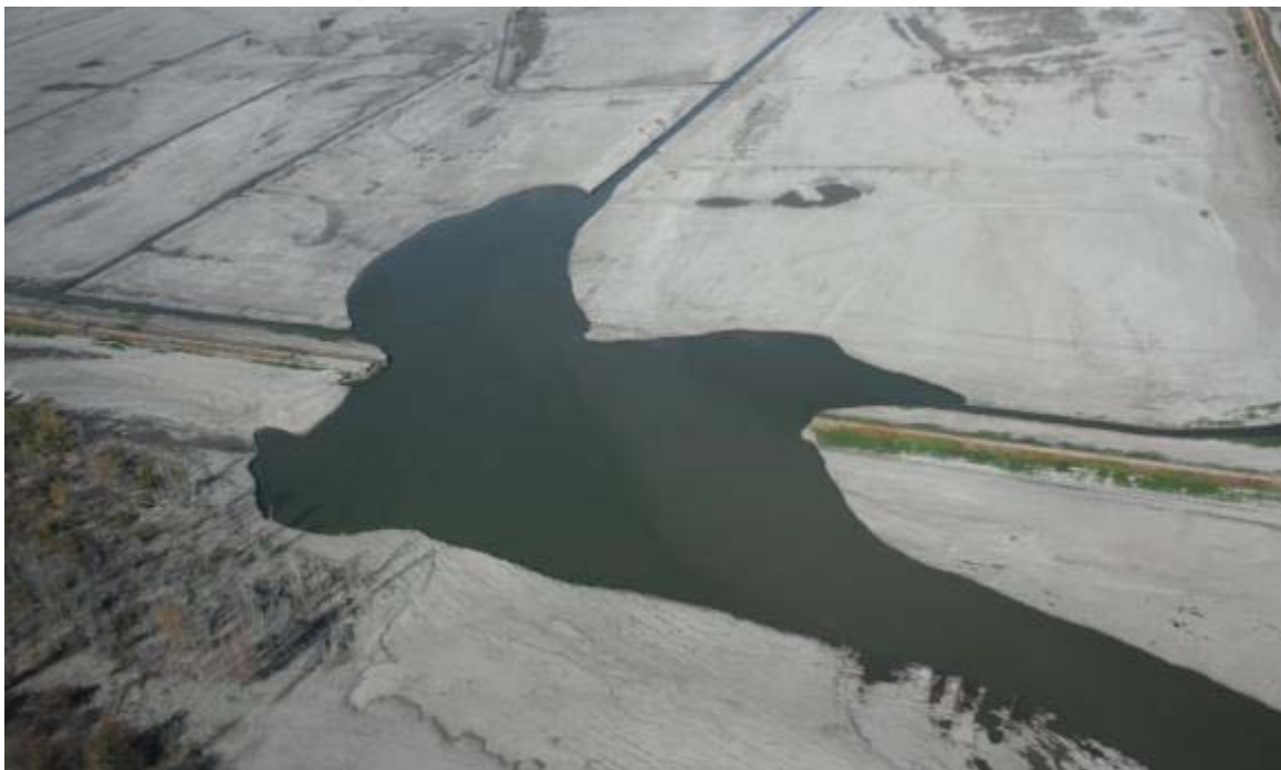
Figure 112. Levee breach: Lower breach at L550
