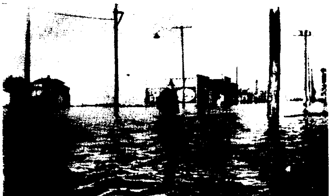
Figure 5. December 1921 Flooding of Skagit River at Intersection of Fairhaven Avenue and Anacortes Street in Burlington.
