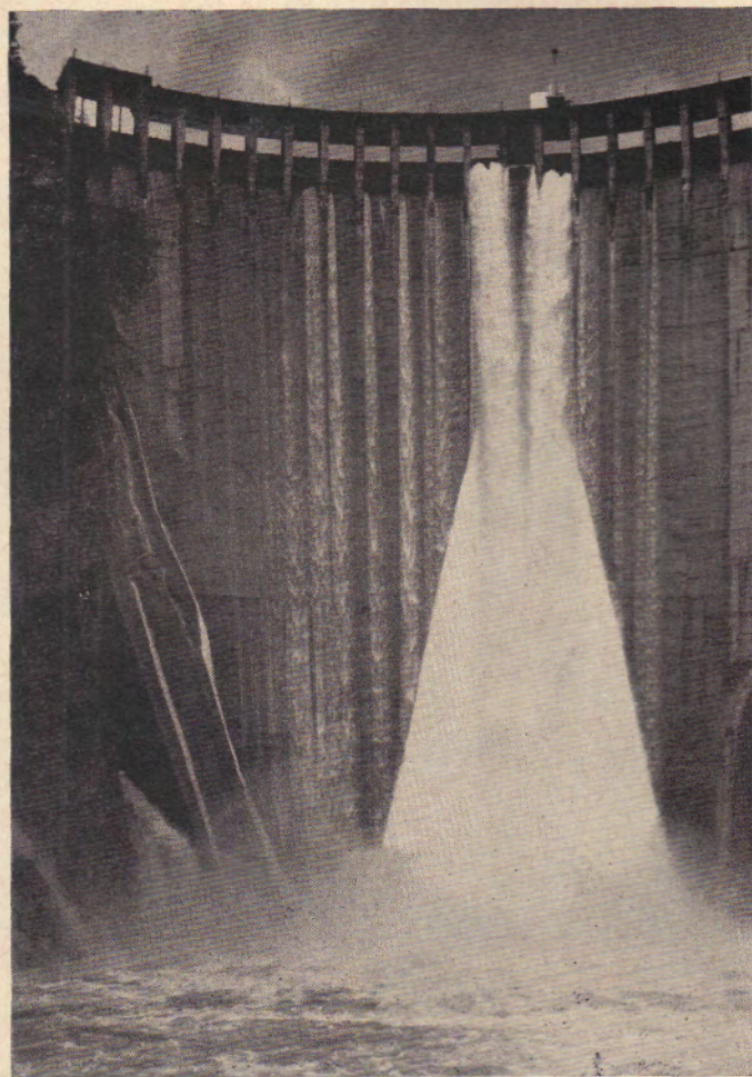
FIGURE 17. Flow over the spillway at Baker Dam with one gate fully open and adjacent gates cracked one foot.
