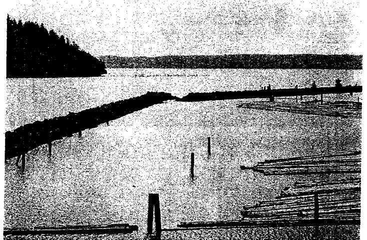
Right — View of the long rock jetty barrier to salmon runs of Swinomish Channel, with the break for the inadequate fishway shown in the center.
