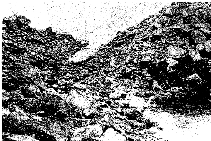
Left — Salmon would have to be flying fish to get through the jetty fishway at low tide. The rock bottom of the fishway is completely exposed at low tide.
