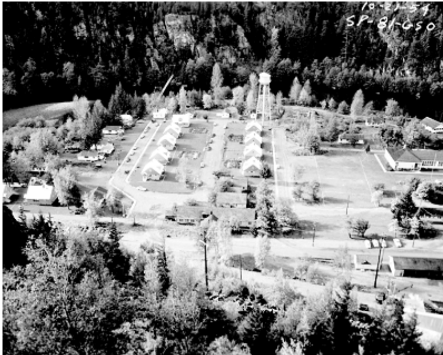
Description: General view of Reflector Bar. Date: Oct 21, 1954 (Source: Seattle City Light. )
