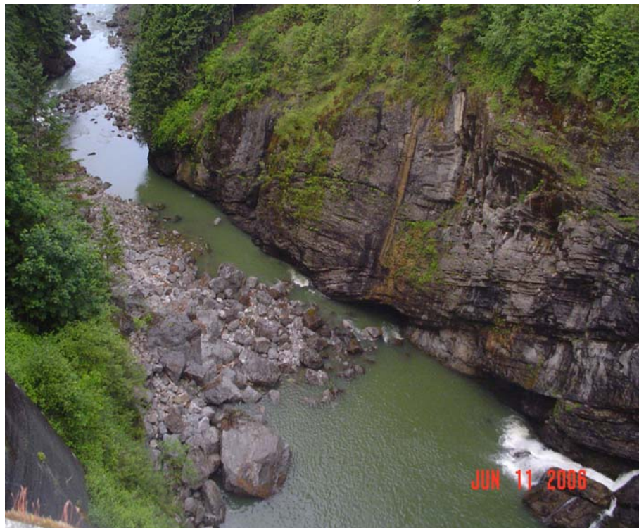
Lower Baker River Canyon (note rockslide)
