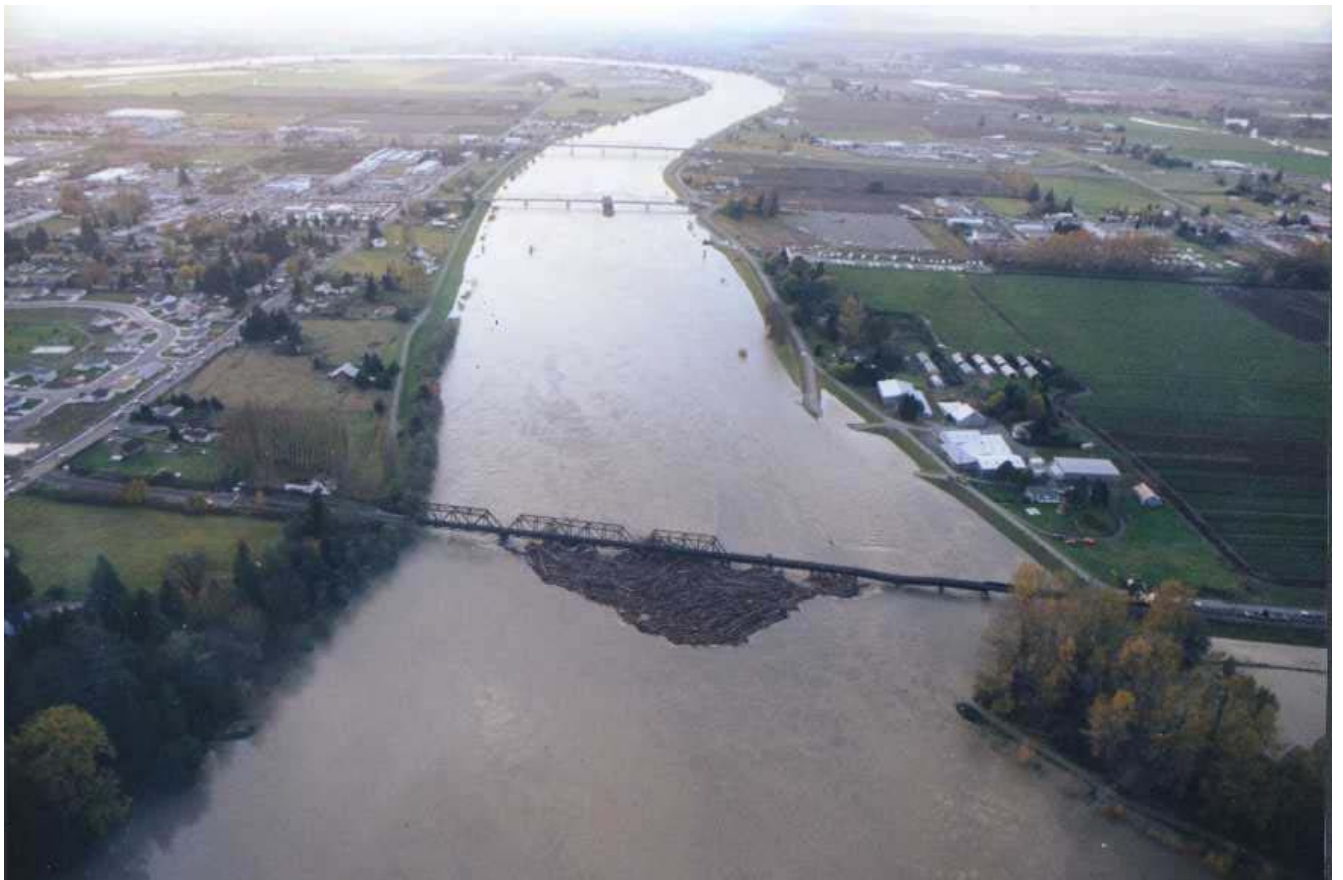
Log jam on BNSF bridge, 1995 flood event. (Source: Corps of Engineers, Seattle District, 1995)
