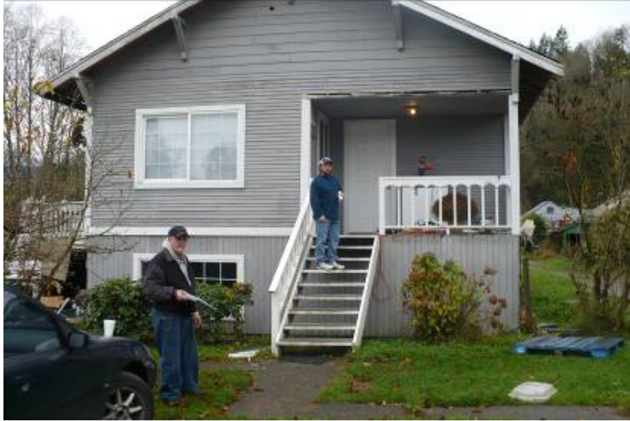
7752 S. Dillard Avenue – Tax Assessor Records Built 1915
