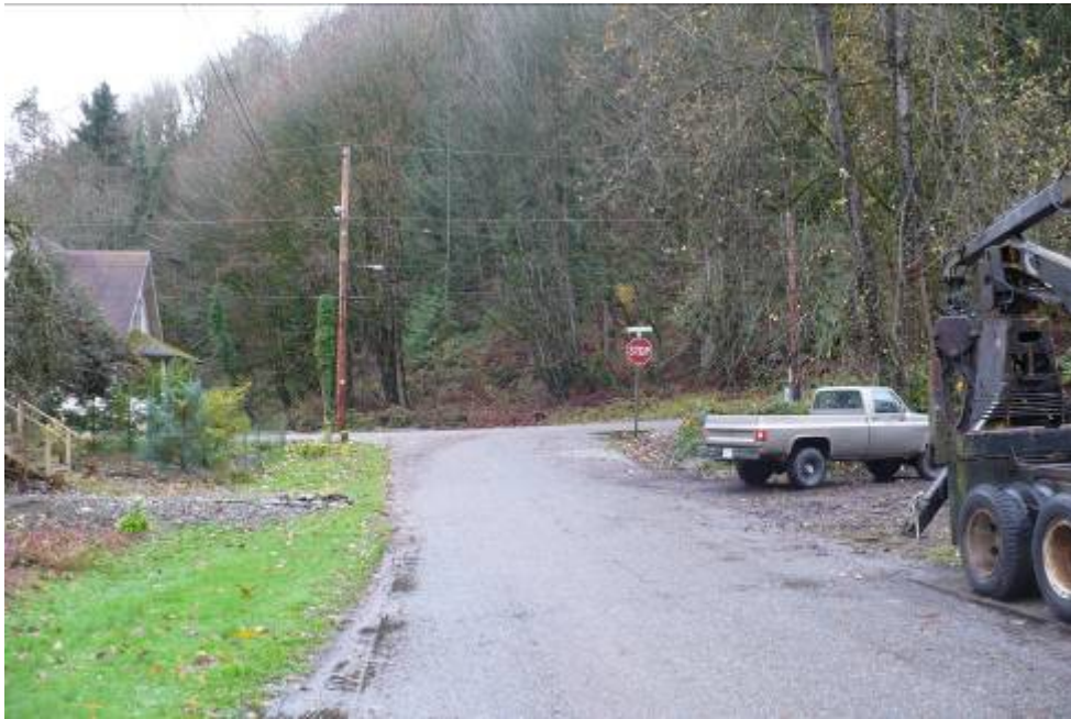
Floodwaters in 2003 made it to base of Stop Sign post.
