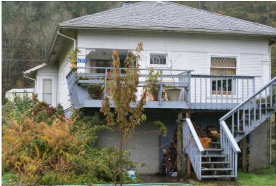
46303 Forest Place – Constructed 1912
