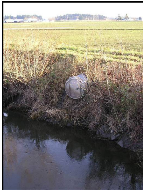
Figure 1-2. Floodgate, Drainage District 25 – Samish River system.
