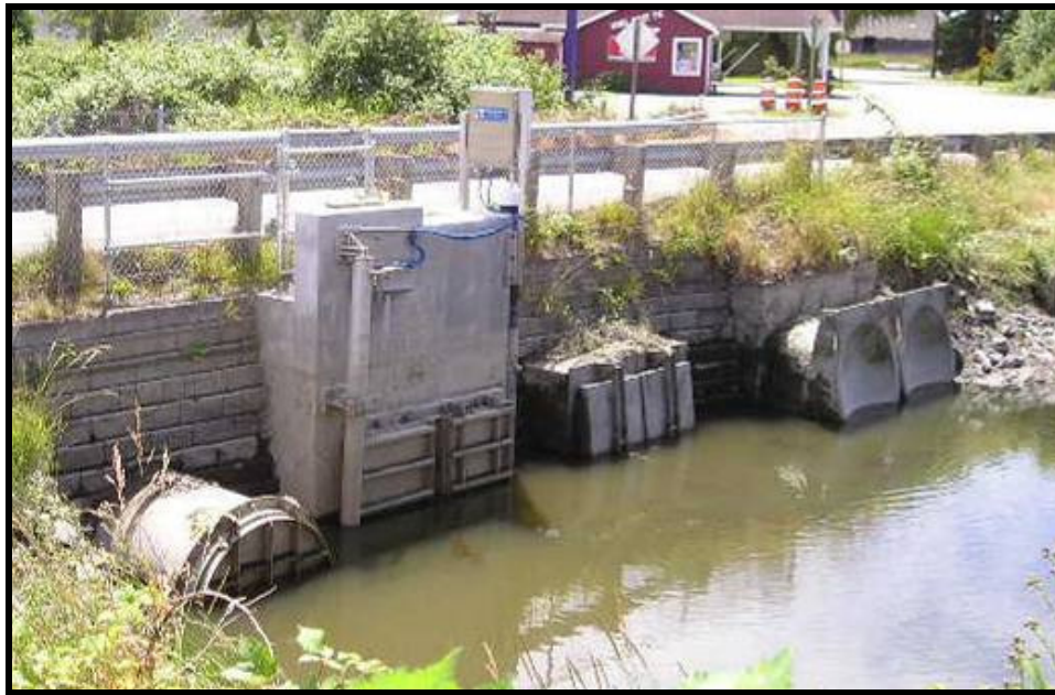
Figure 1-1. Tidegates on Edison Slough, various top-hinged gates and a Self Regulating Tidegate (center left). County maintained tidegate complex.
