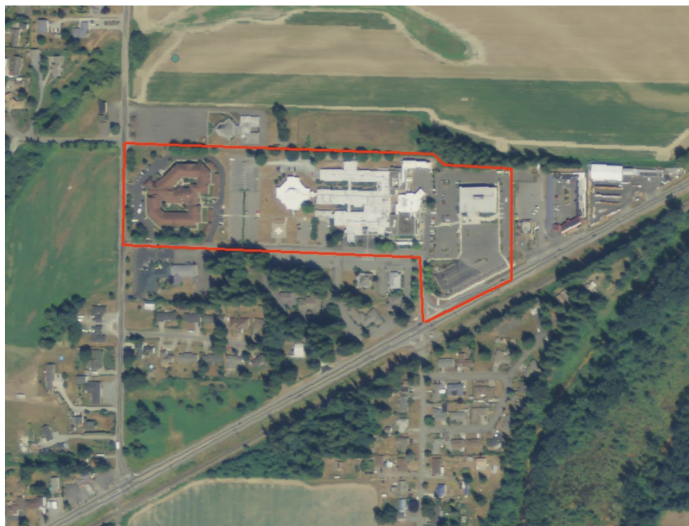
Figure 33: United General Hospital facility levee
