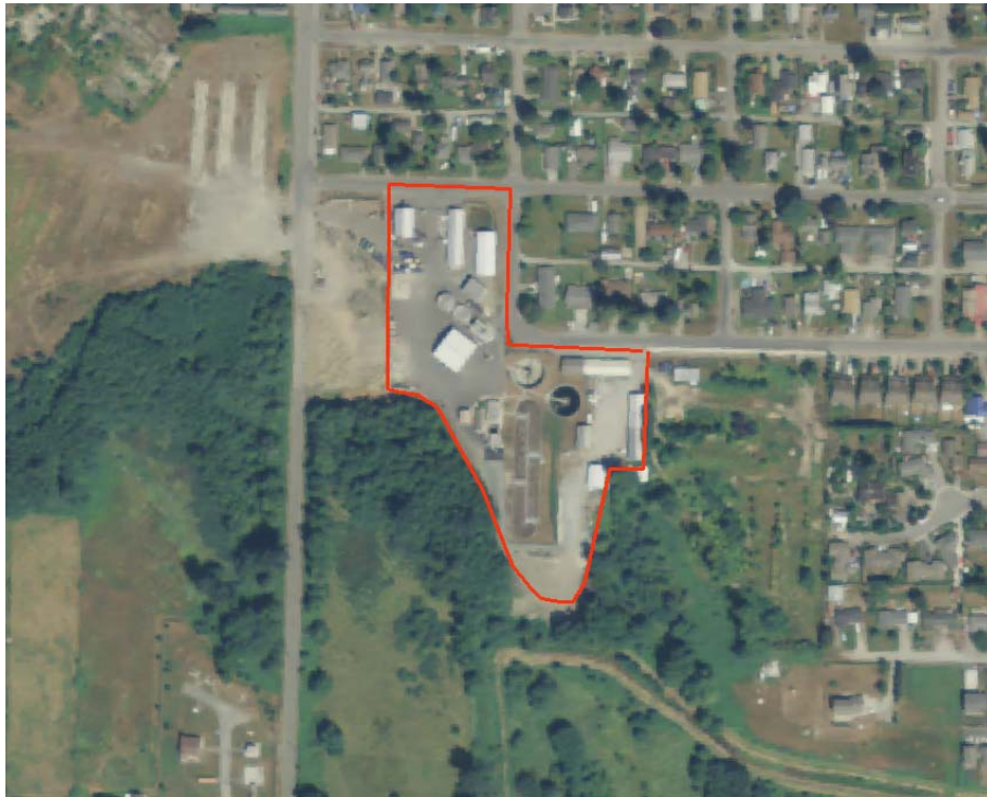
Figure 37: Sedro-Woolley Waste Water Treatment Plant facility levee
