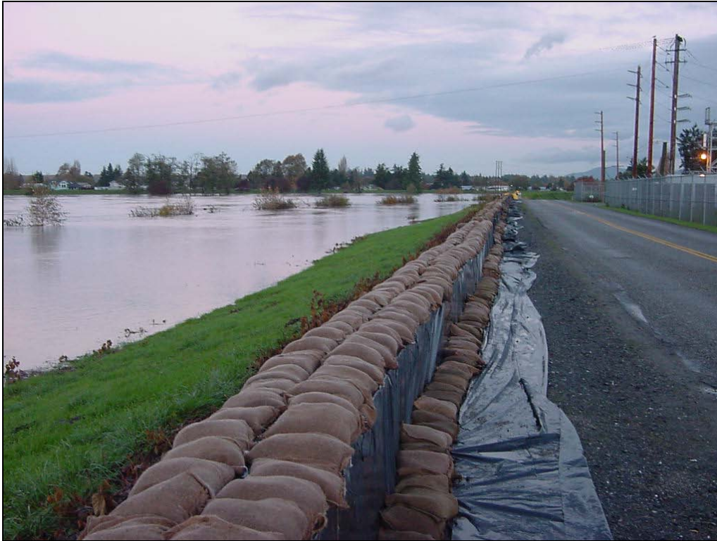
Flood Fighting Efforts to Save Water Treatment Plant (Courtesy of Willy LaRue, City of Anacortes, WA)
