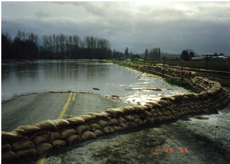
Sandbagging along Whitmarsh Road, Burlington, WA (Courtesy of Dike District 12)
