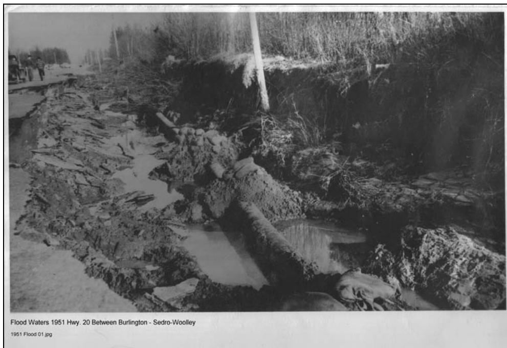
1951 Flood Damage between Burlington & Sedro-Woolley on Highway 20 (Courtesy of Roger Fox Collection)
