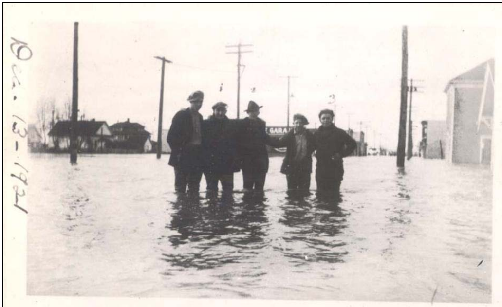
Fairhaven Avenue, Burlington, WA – Looking West (12/13/21) (Courtesy of U.S. Army Corps of Engineers)
