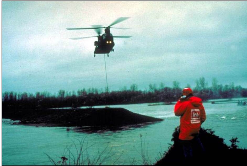
Levee Break on Fir Island (2001) (Courtesy of U.S Army Corps of Engineers)
