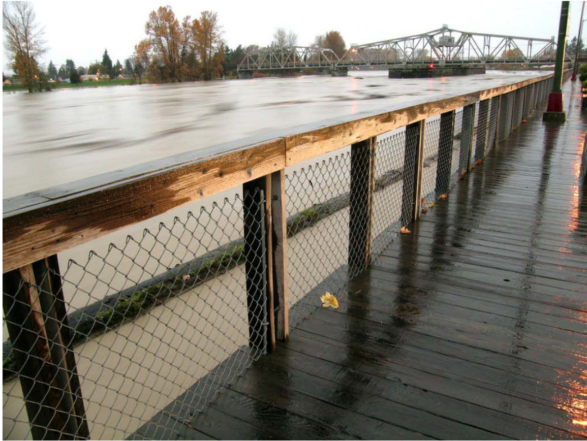
Water Reaching The Revetment
