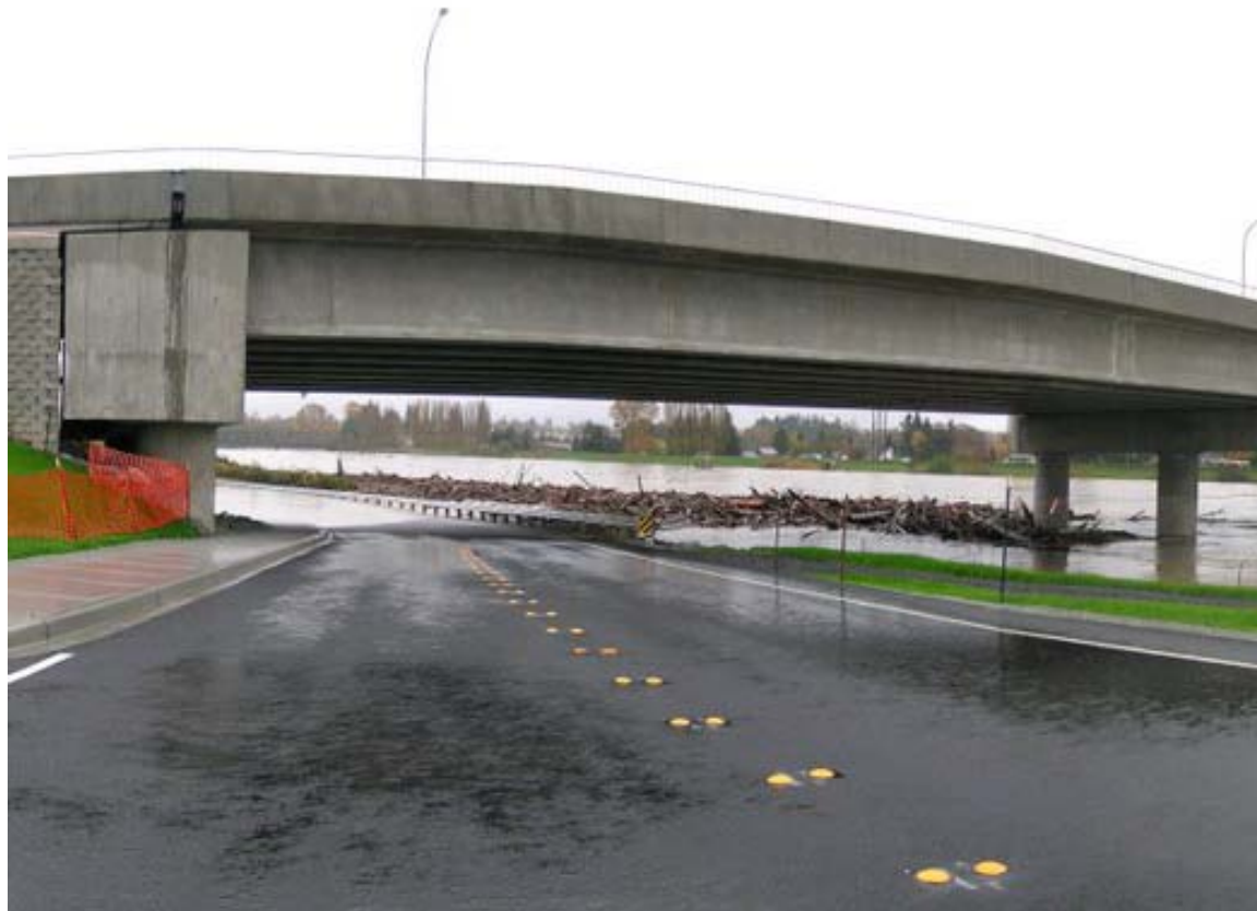
Flooding Under New "Old 99" Bridge
