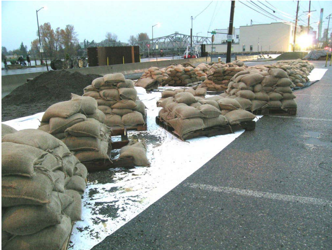
Sandbagging and Staging Along Revetment
