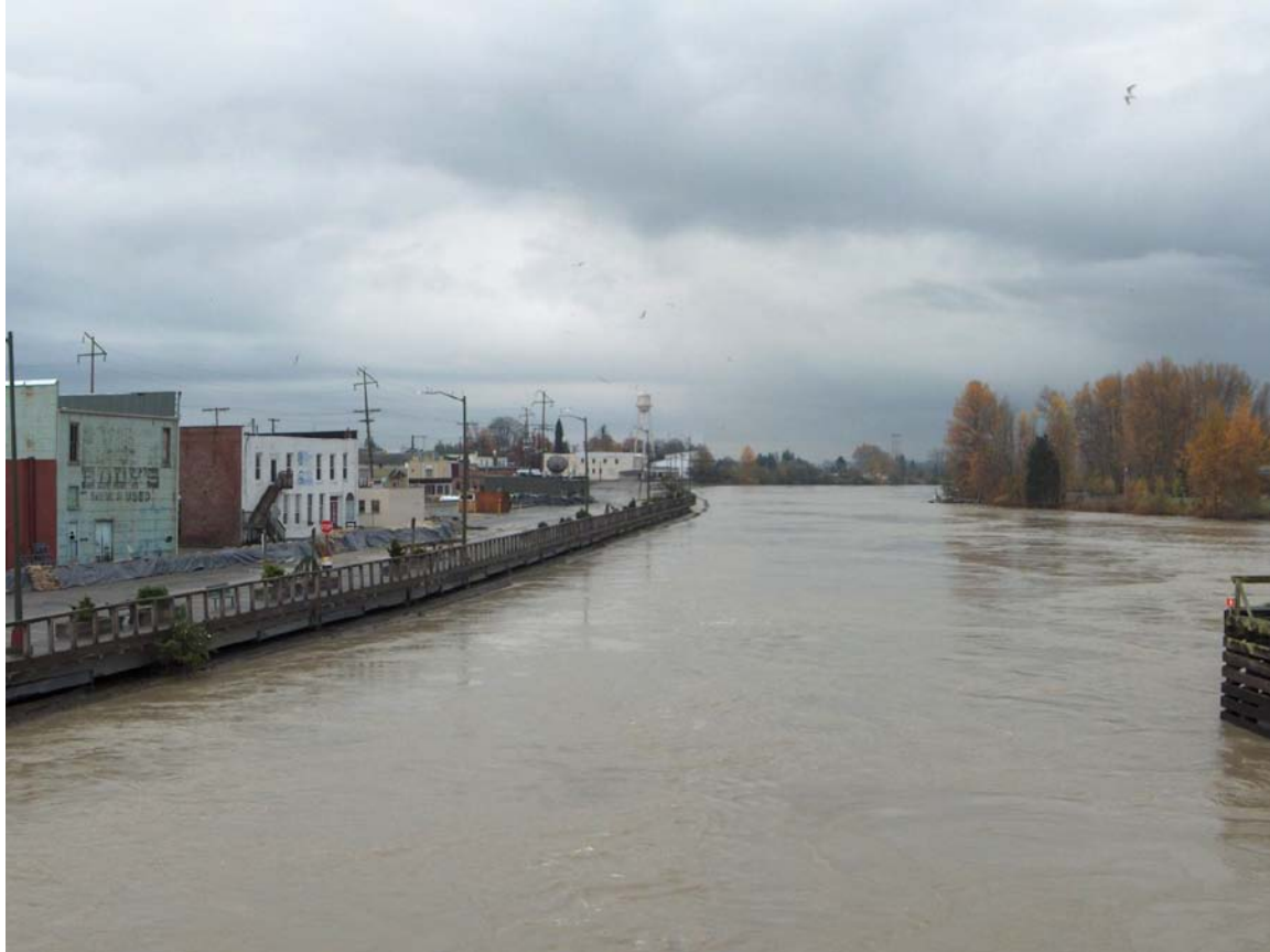
Photo From West Mount Vernon Bridge
