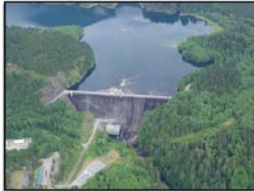
Upper Baker Dam
