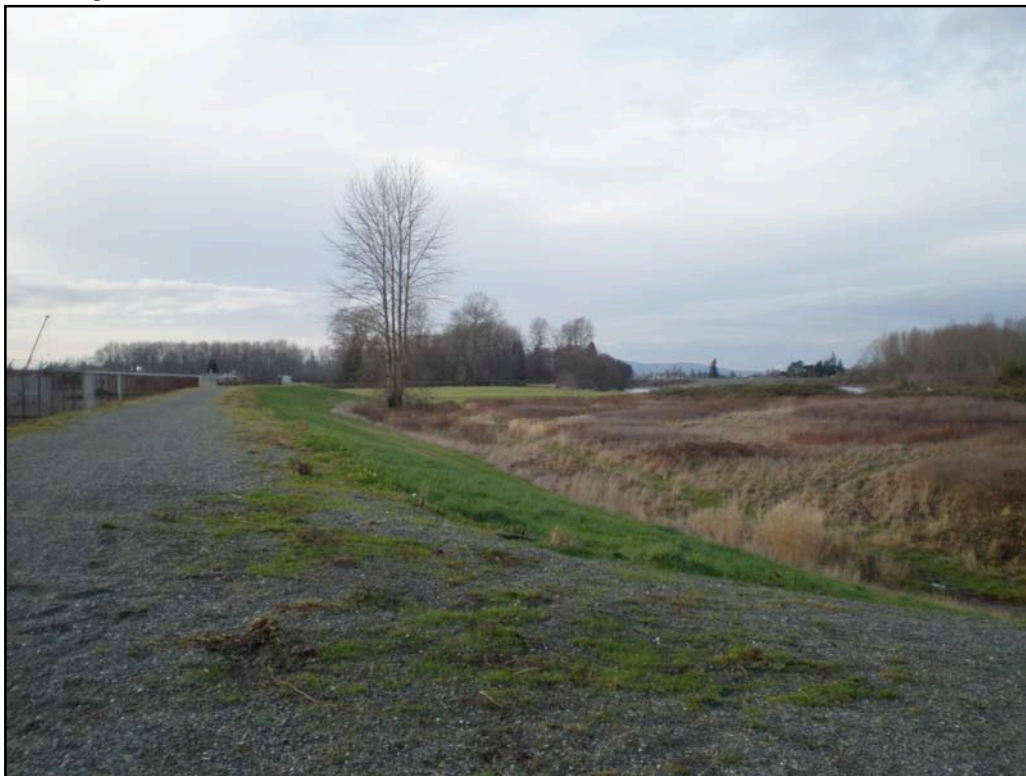
Figure 11. Existing levee north of the WWTP in the southwestern portion of the APE.
