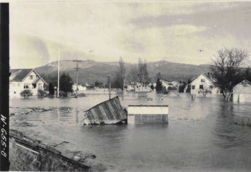
A few small buildings were moved by the flood at Conway. Many older homes in this area had first floors above the water line. Lack of electric power and domestic water supply added to the inconveniences caused by the flood.
