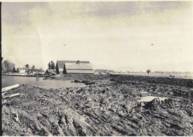
Looking northeast toward Boswyk farmstead on Fir Island, showing new dike construction. Old dike in left along with granary was completely washed out when flood waters from Dry Slough break swept down to lower end of diking district.
