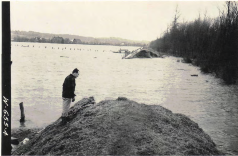
At Conway the dike on the east side of the South Fork of the Skagit river broke, inundating an area extending from approximately one mile south of Mount Vernon to an area south of Stanwood in Snohomish county. More than 250 Skagit county homes were damaged to an extent of $500,000 as a result of the high water.
