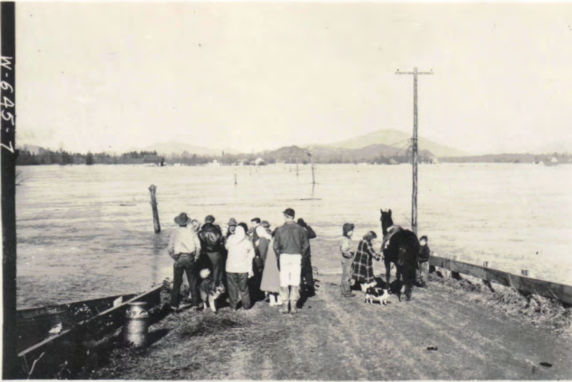
Looking north down County highway in Nookachamps area three miles northeast of Mount Vernon. This undiked area provides a flood basin for the Skagit river at high water. Road was inundated to a depth of eight to ten feet.
