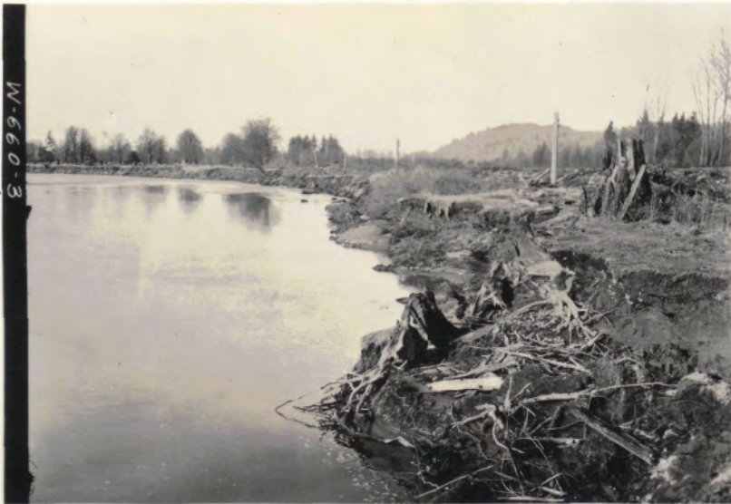
The Skagit river above Sedro Woolley did extensive stream-bank damage at many places and the deposition of sand and debris resulted in substantial channel changes at many points.
