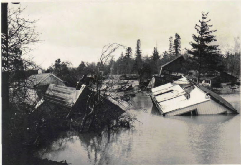
At the Moore farm the water destroyed the house, barn and machine shed. Parts of these buildings were carried away as swirling waters cut into the subsoil.
