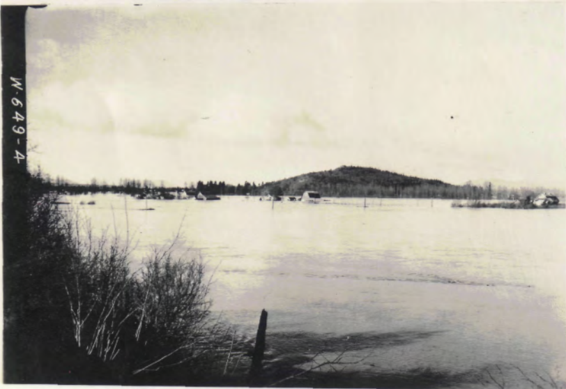
Looking northwest across Nookachamps basin toward Burlington hill. Continuing high water completely filled this storage basin, causing lower river to rise higher than the 1949 flood.
