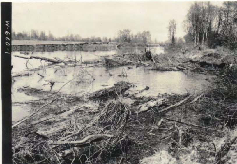
The Dry Slough dike break released Skagit River water to the western part of Fir Island, covering the area between Dry Slough and Deer Slough with many feet of water. The break cut a new channel through the Lee and Tellesbo properties, making many acres unfit for further agricultural use. Deposits of coarse sand caused additional damage.
