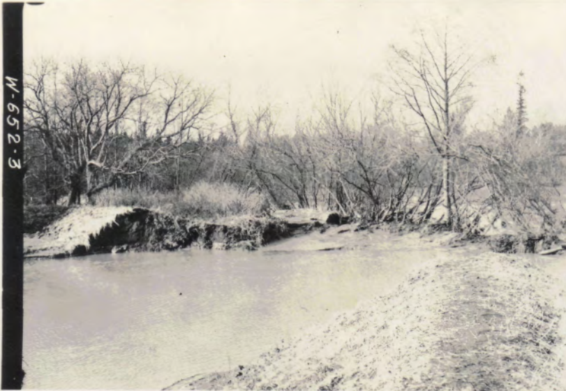
Dikes along the Skagit river from Burlington to the mouth of the river were severely taxed at many points. Emergency sandbagging prevented many breaks. The Moore dike break below the North Fork bridge flooded the west half of Fir Island.
