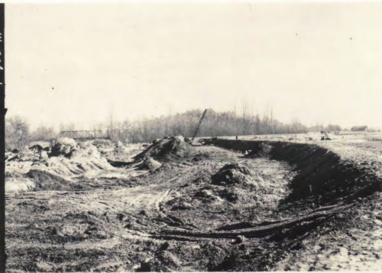
County and State work together to restore dike near Moore Slough break at North Fork bridge. Temporary dike in right of picture which is 950 feet long was constructed in 15 days with use of dragline. Temporary dike will be raised and widened to form permanent structure. Moore farmstead in left will be outside new dike.
