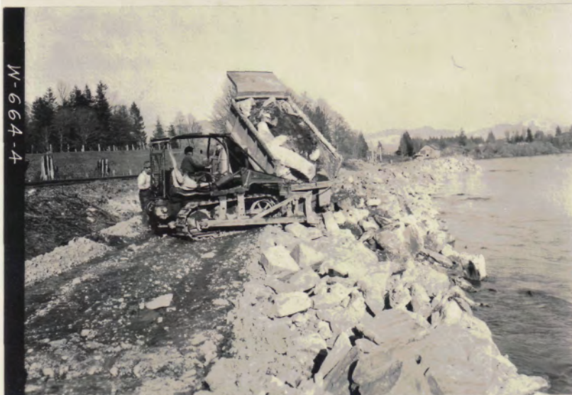
By March 19th the Great Northern Railroad had almost completed revetting the river bank with heavy rock in order to protect the railroad.
