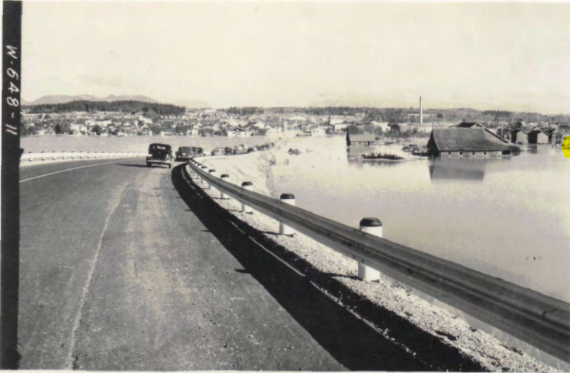
Skagit river flood water did extensive damage in the Stanwood area five miles south of the Skagit County line. Looking east toward Stanwood and East Stanwood from Camano Island viaduct, showing extensive damage to farmsteads, business and residential property.
