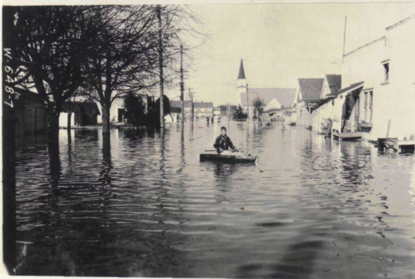
Looking up Stanwood street showing high water.
