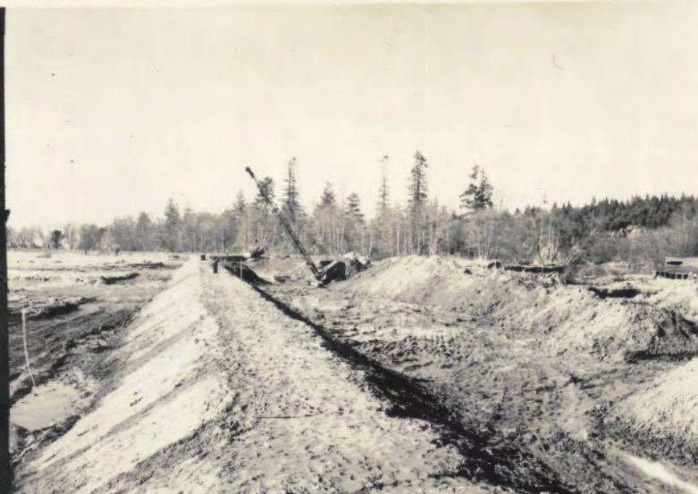
Looking southwest across temporary dike at Moore break being constructed through cooperation of State and County. Skagit river channel through trees in background.
