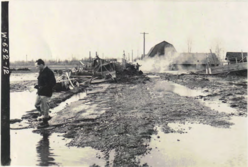
Looking west down County road past Noble Lee farm. County equipment is clearing debris including transient labor tent houses from road.
