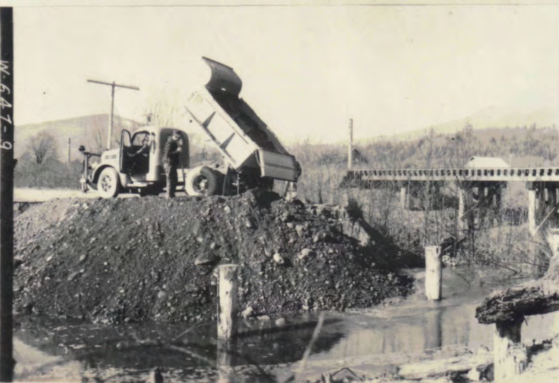
The State highway between Hamilton and Concrete was completely washed out at a point two miles east of Hamilton. Access to points up-river was possible through the use of Sound View Logging Company road from Hamilton to Grandy Creek near Birdsview.
