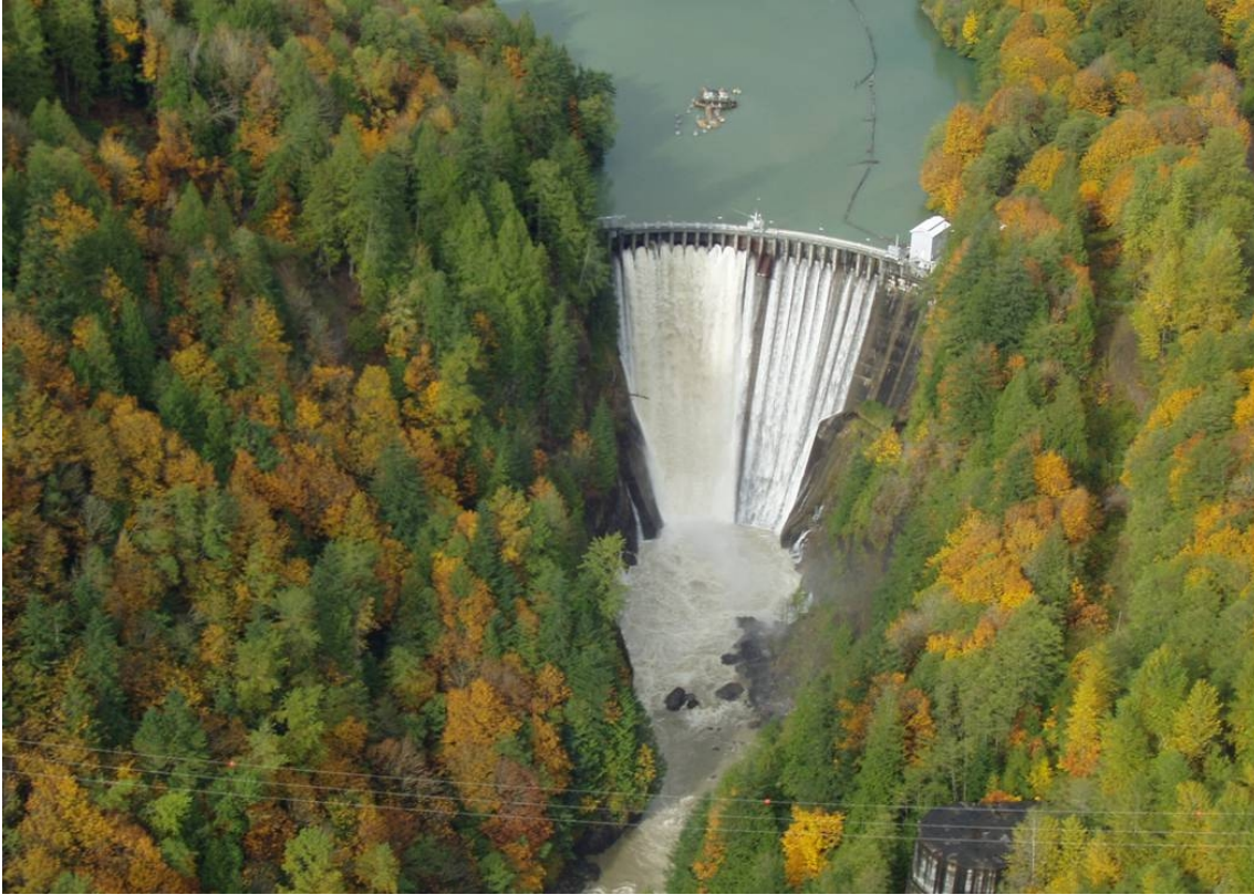
Figure 4 Lower Baker Dam spillway discharge evacuating Lake Shannon
