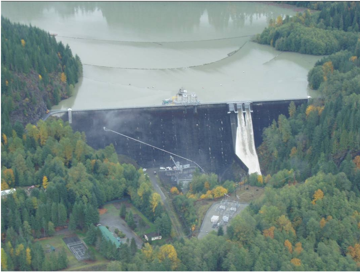
Figure 2 Upper Baker Dam spillway evacuating Baker Lake
