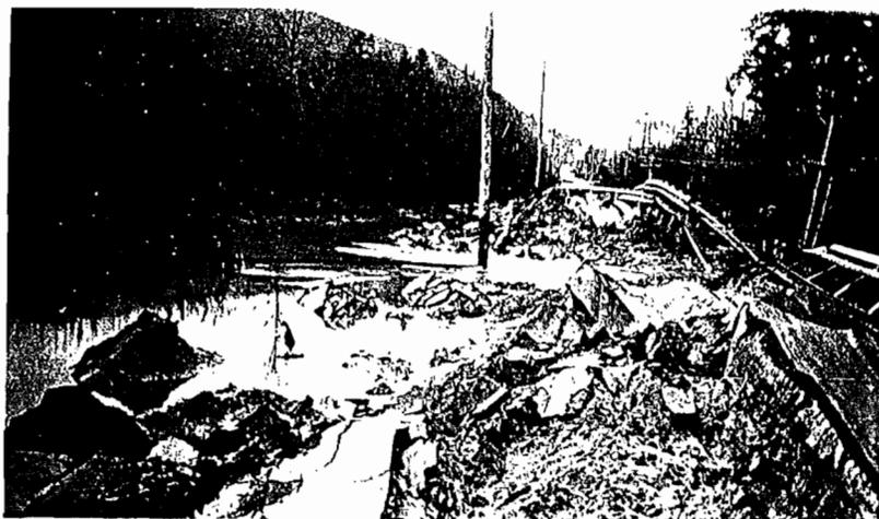
No. 2. Looking south along the Clear Lake road from near the city limits of Sedro Woolley. This fill was composed of sand with some clay and flattened out like molasses when it became saturated. The fill was not overtopped. Note some water still flowing through the break. Picture taken 10:00 a.m., Feb. 29.
