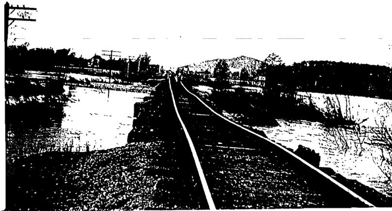
No. 16. Looking north along the Great Northern Railway washout, near Burlington. Track undermined for 360 feet at this location. A break occurred here during the 1921 flood. Note that the old trestle used in repairing the roadbed after the 1921 flood is still in place and was used to shore up the track after the present flood. Picture taken at 2:00 p.m., Feb. 29th.
