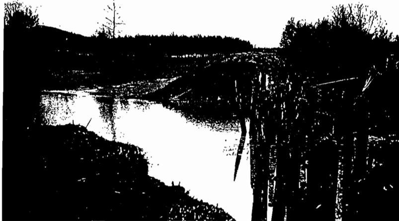
No. 7. Looking upstream (north) along the broken dike above the Great Northern Railway bridge. (mile 16.2). Note the old pile trestle that was used to repair the dike after the 1921 flood. The main river channel is on the right. Picture taken 2:00 p.m., March 1st.
