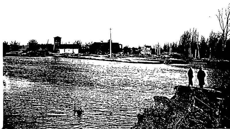
No. 10. Looking upstream along the dike at the break on the right bank of the South Fork a mile north of Conway, taken about 2:00 p.m., March 2d. The river channel to the right is not visible. The lake in the foreground is formed by the water after passing through the broken dike. Note the numerous large snags stranded in the door-yard. The white house in the left background was knocked off its foundation.
