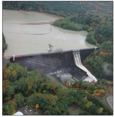
contribution to the 100-year flow is 9,000 cfs which represents 4% of the total flow. These measures are designed to reduce the flow contribution coming from Upper Baker Dam with additional storage, timing, and minimum outflow adjustments.
