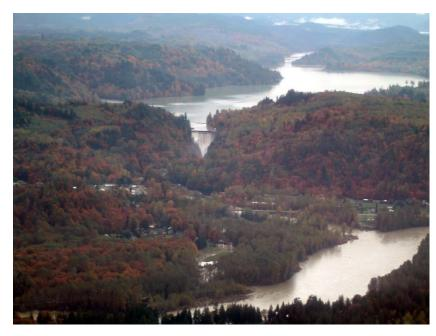
With the existing flood control space and flow releases at Upper Baker Dam, Lower Baker Dam's combined existing outflow contribution to the 100-year flow is 16,500 cfs which represents 7.3% of the total flow (7,500 cfs is the runoff between Upper and Lower Baker Dam and 9,000 cfs is the release from Upper Baker). These measures are designed to reduce the flow contribution coming from Lower Baker Dam with storage and outflow adjustments.
