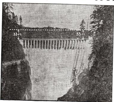
With 33 feet added to the height of the Baker River Dam at Concrete for the Puget Sound Power & Light Company the great structure will be 293 feet high, practically doubling the water storage capacity.
