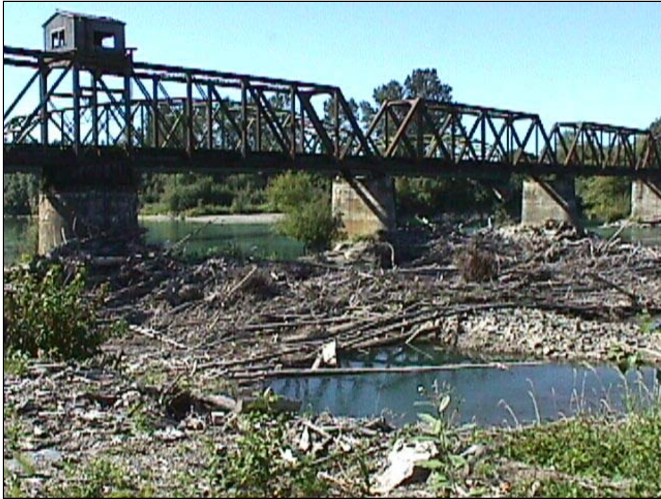
BNSF Railroad Bridge Log Jam, Burlington, WA (1999) (Courtesy of Skagit County Public Works)
