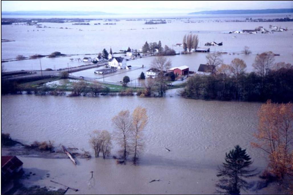
Levee Break at Fir Island, Mount Vernon, WA (2001) (Courtesy of Skagit County Public Works)
