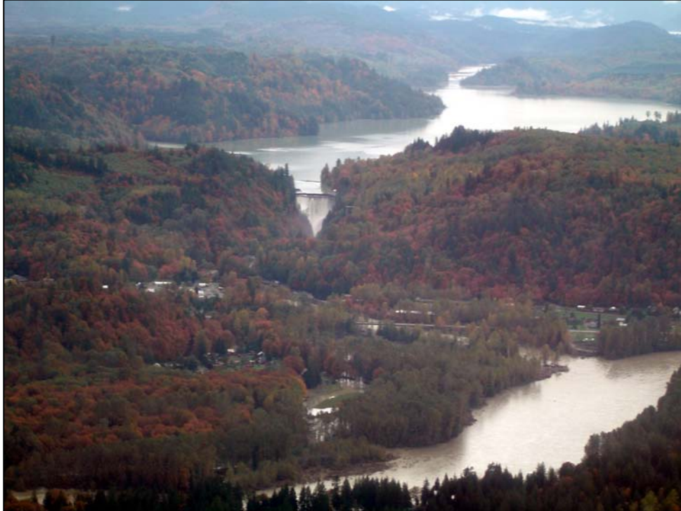
Lower Baker River Dam (Courtesy of U.S. Army Corps of Engineers)
