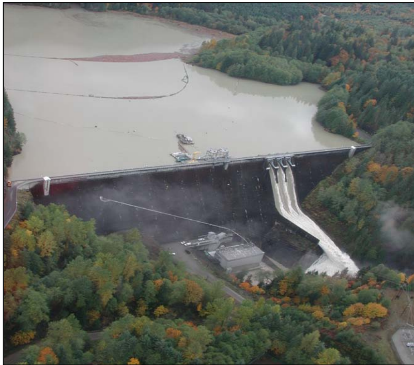
Upper Baker River Dam (Courtesy of U.S. Army Corps of Engineers)
