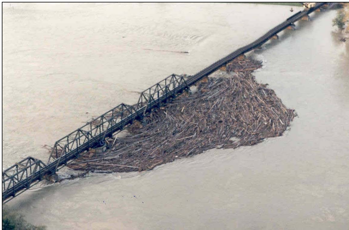
Burlington Northern Santa Fe Bridge (1995) (Courtesy of the U.S. Army Corps of Engineers)
